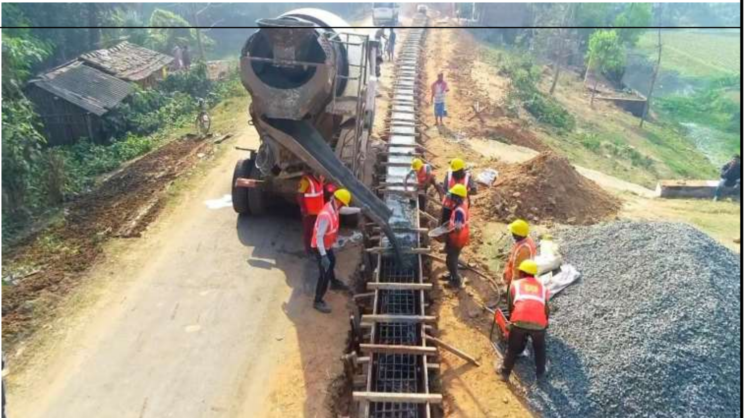
Completed 0.5m Flood Wall Ch. 32500m (PKG-I)
