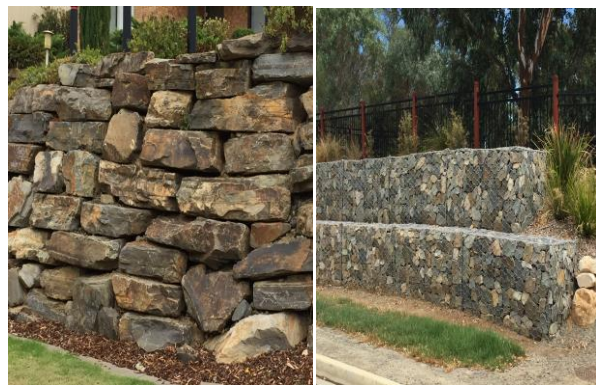
Alternative materials, left quarry stone and right gabion- photo credit Mike Williams
