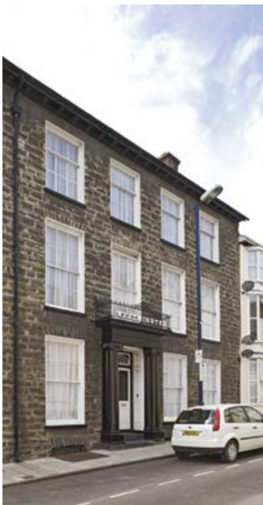
Built for the Pughs of Abermad, this house was one of several gentry houses on Bridge Street, a fashionable residential street in the early nineteenth century (Crown Copyright: RCAHMW).
