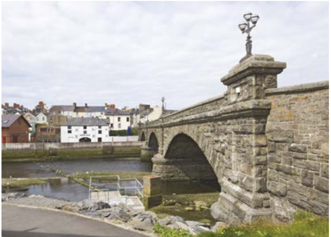
The late nineteenth-century bridge at Trefechan and a former corn-store — a rare survivor of a harbour-side warehouse (Crown Copyright: RCAHMMW).
