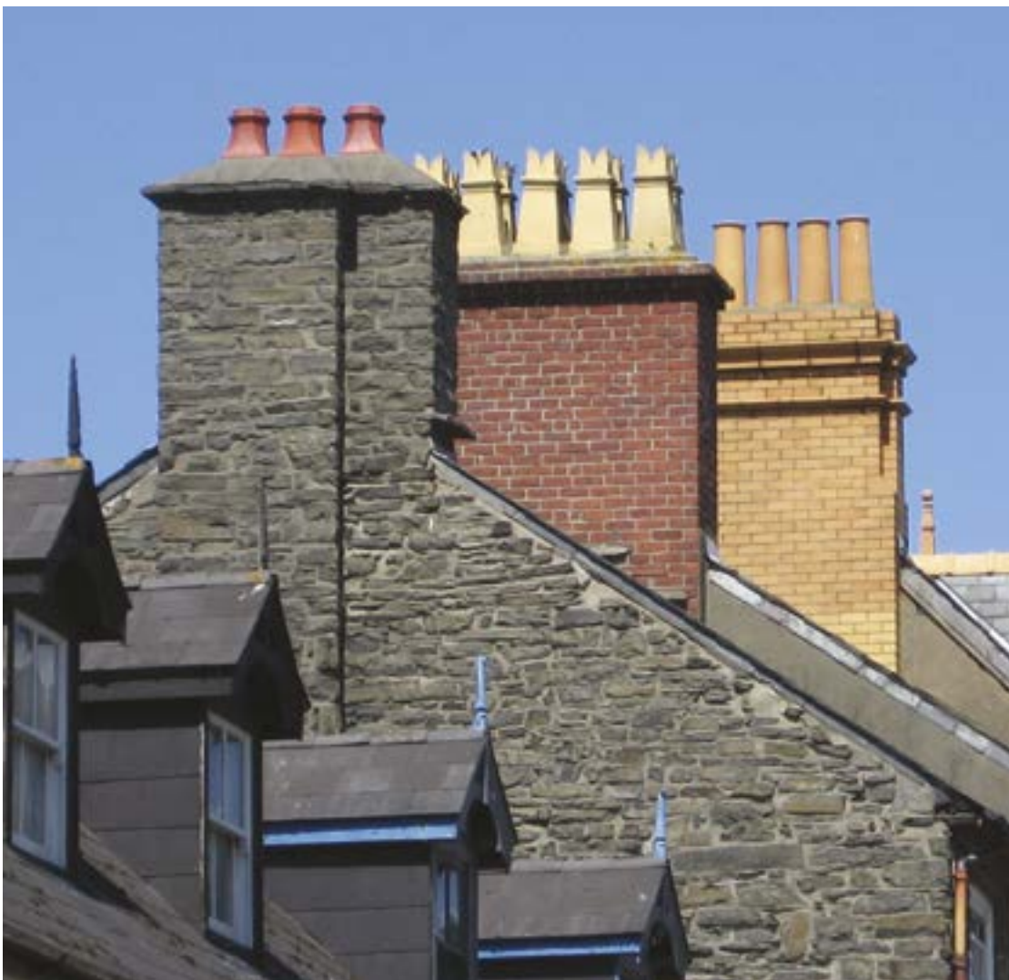
Chimneys are an important aspect of the roofscape (Crown Copyright: Cadw).
