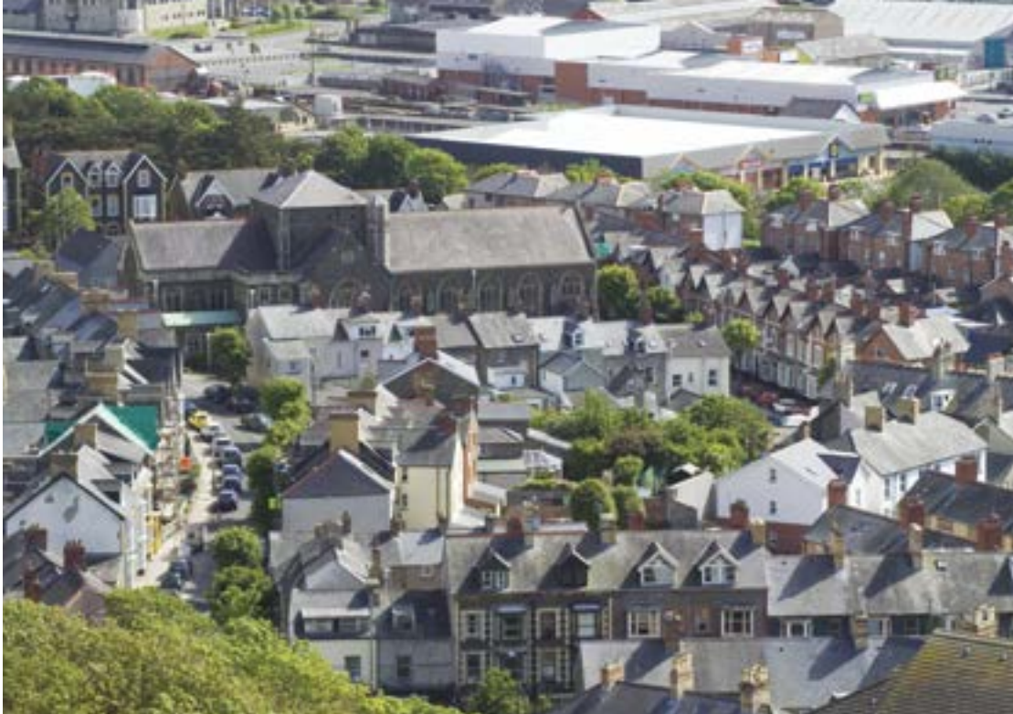
The parish church of the Holy Trinity forms an architectural anchorage for The Buarth (Crown Copyright: RCAHMW).
