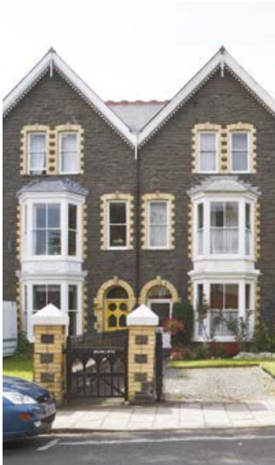
Far right: An unusual porch on Llanbadarn Road (Crown Copyright: RCAHMW).
