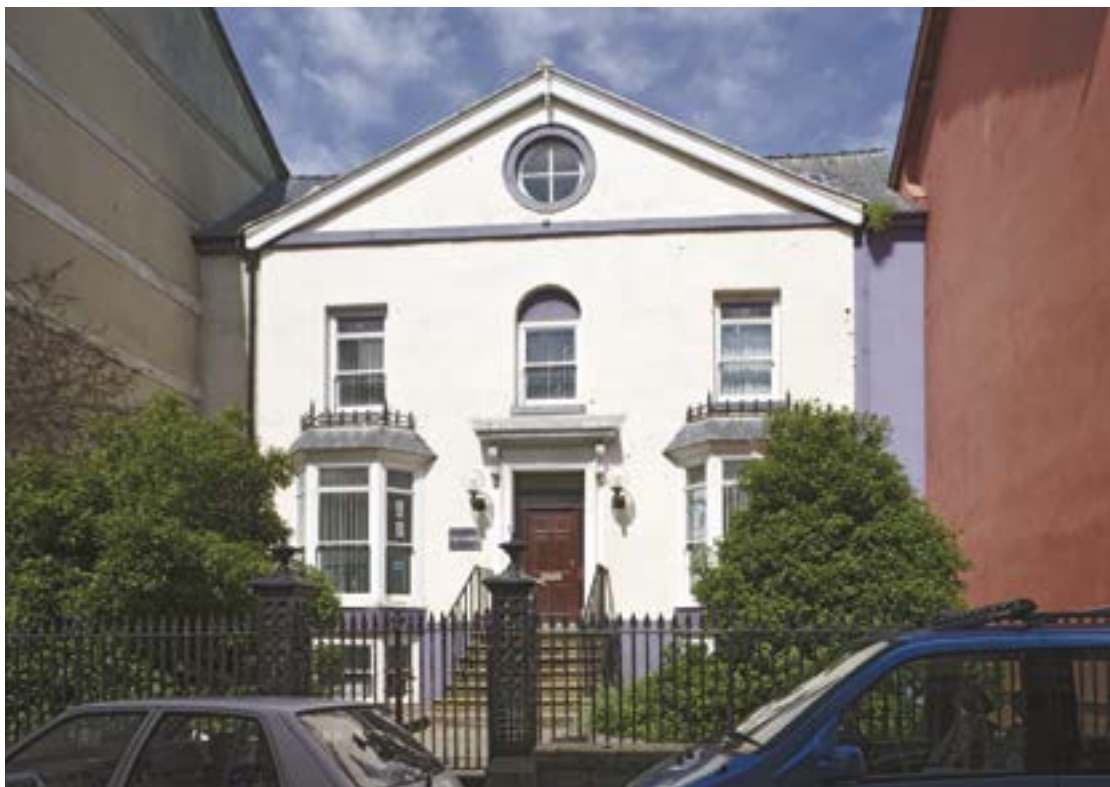
Crynfryn House on Eastgate was the town house of the Bonsall family, before it became a hospital in the mid-nineteenth century (Crown Copyright: RCAHMW).
