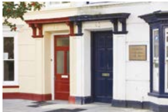
Left: Doorcases and doors on Portland Street (Crown Copyright: RCAHMW).
