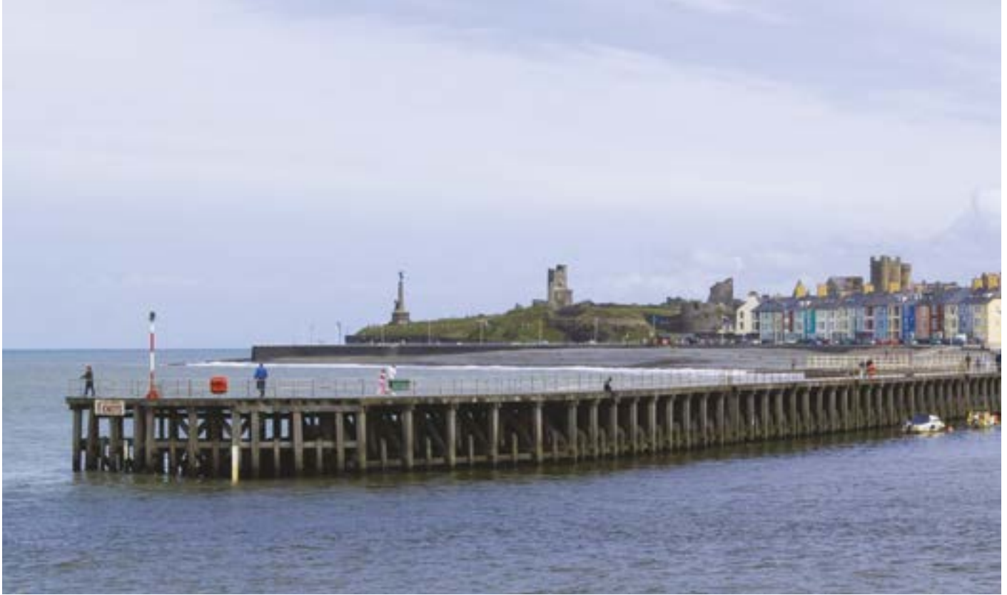
Above: The wharves and quay wall on the west side of the harbour were first built in 1858 (Crown Copyright: RCAHMW).
