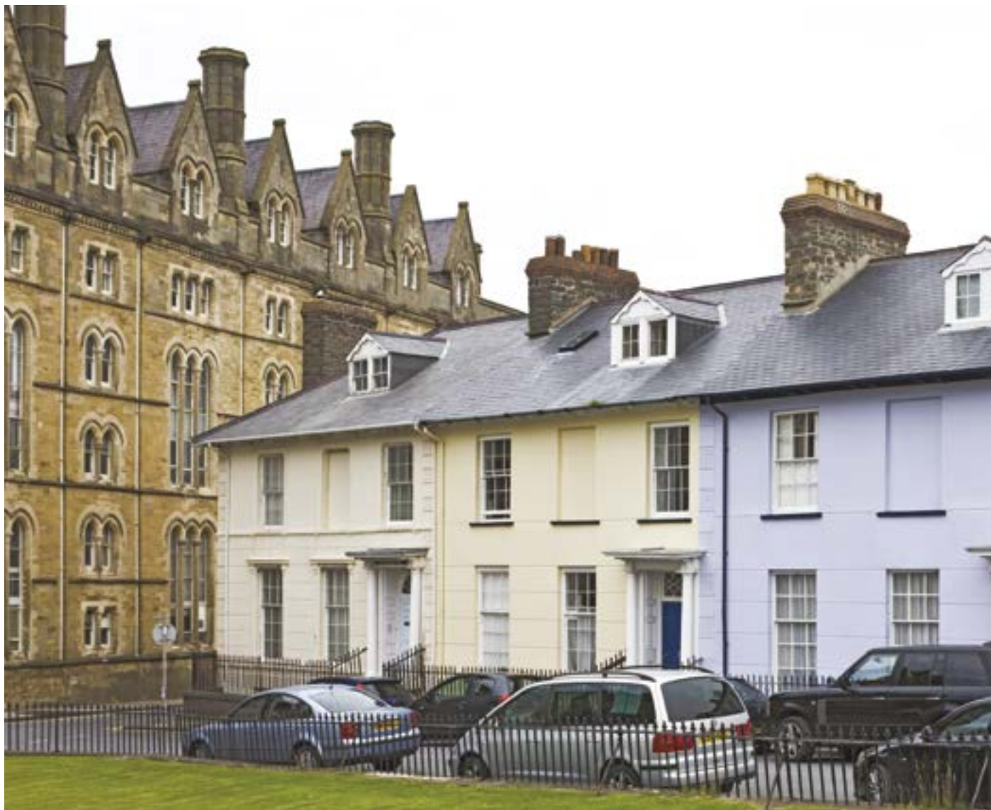
Contrasting styles: Old College and the houses of Laura Place (Crown Copyright: RCAHMW).
