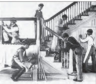
Carpentry students learning how to construct a staircase
