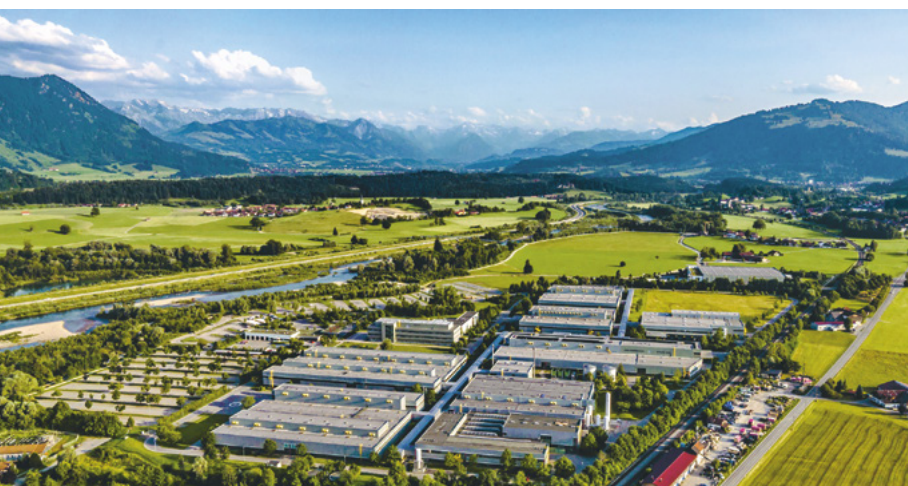
The Bosch site in Blaichach, Germany, relies on smart energy management
