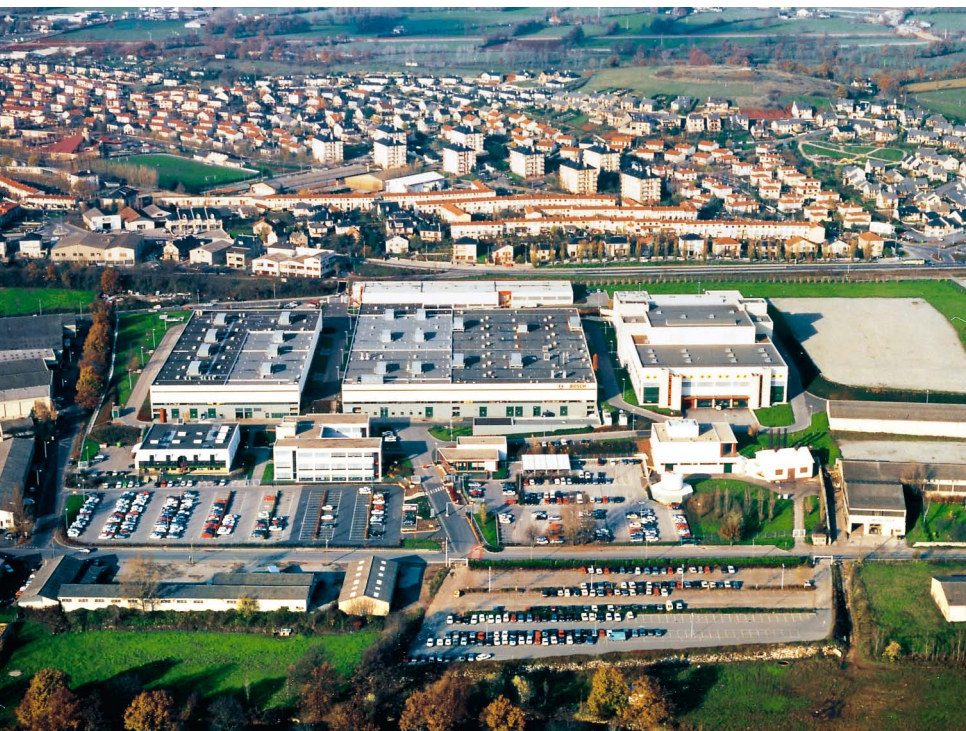
On average, 90 percent of the heating requirements at the Bosch location in Rodez, France, are met by its new biomass heating plant
