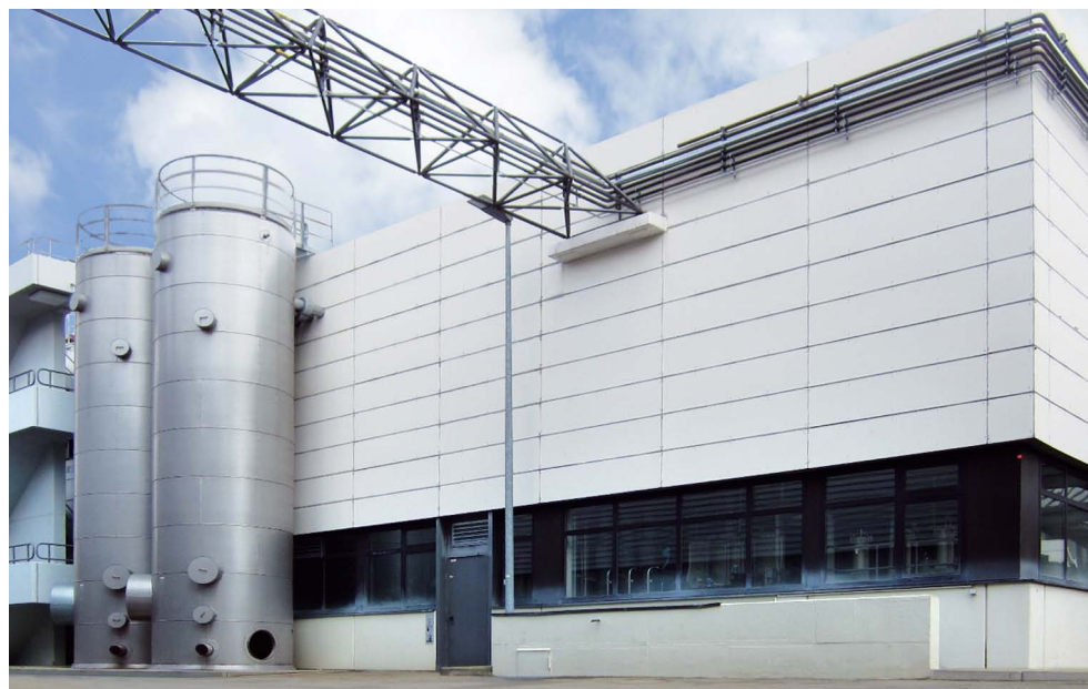
Reutlingen plant uses waste heat from cooling water to reduce its energy consumption
