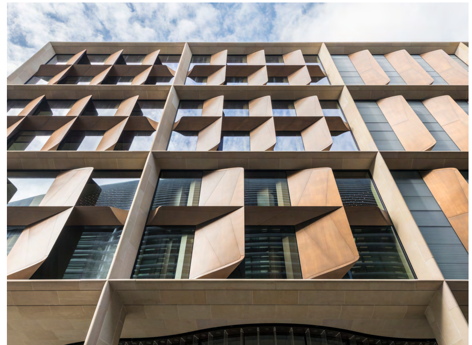
Our London building features bronze window blades that open, allowing us to increase fresh air flowing through the space.
