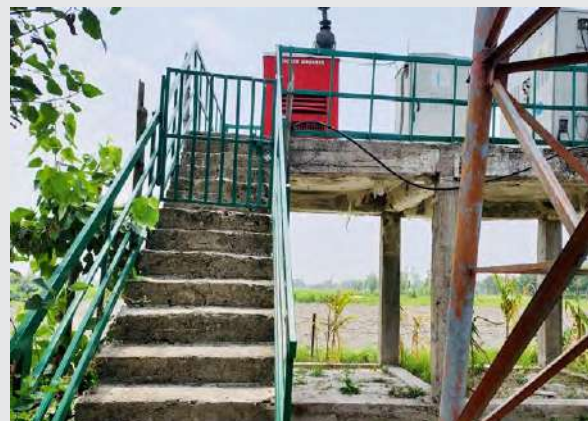
Infrastructure elevated to combat flood impact
