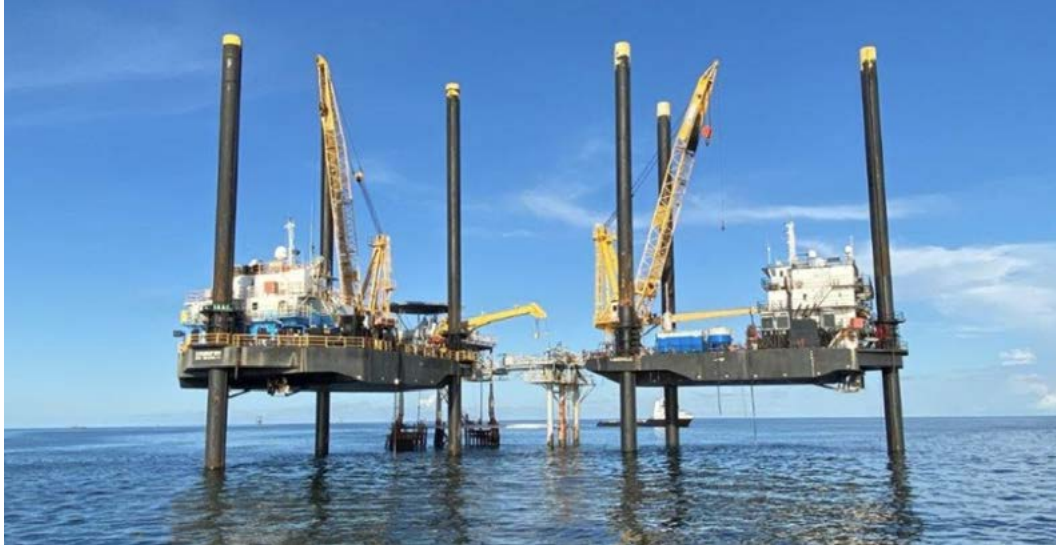
↑ Two liftboats remove an offshore rig platform in the GOM.
