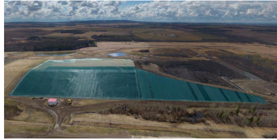
Permanent capping on the left, staged capping in the lower right and an active landfill on the upper right at SECURE's La Glace landfill.
