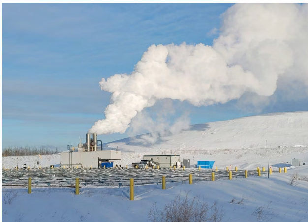
Evaporation unit operating at the South Wapiti Landfill.
