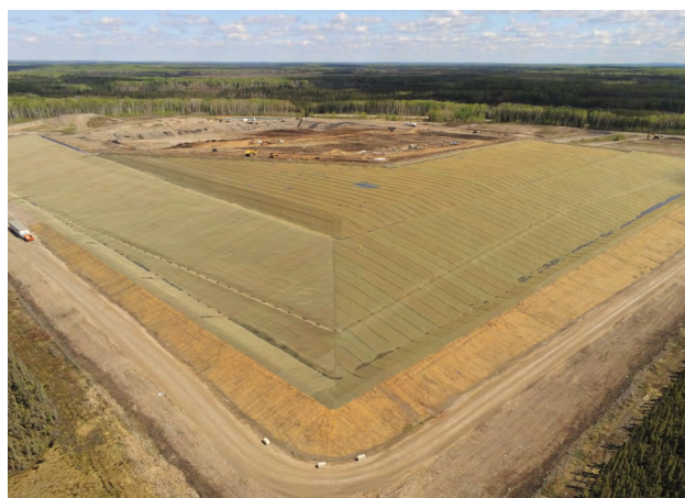
Completed capping at SECURE's Janvier landfill in 2020.
