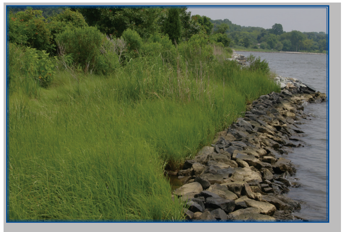
A hybrid solution for this medium energy environment includes a rock toe at the edge. Source: Burke Environmental Associates: http://www.burkeassociates.biz/LivingShorelinesP.php
