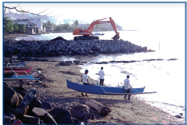
Design of shoreline structures must consider the adjacent shorelines to insure that the erosion is not exacerbated.
