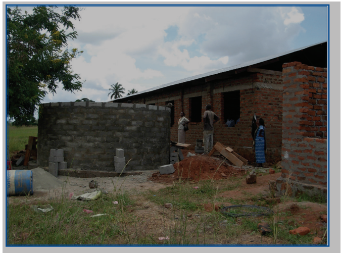
Constructing water tanks for schools in Tanzania's Wawi Watershed is critical to address current climate issues and to improve for health and sanitation of the community.
