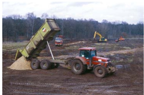
Restoring the Banisveld
