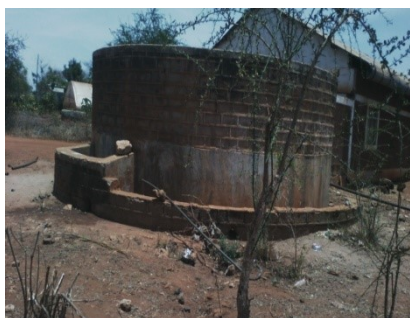
Plate 1: Masonry water tank
