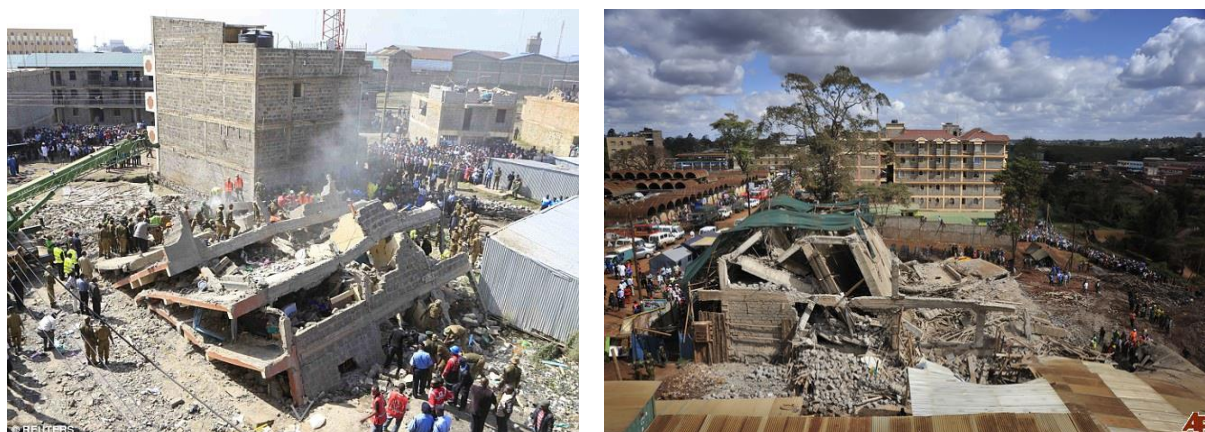
Figure 8: Collapsed buildings in South B, Nairobi and Kiambu respectively
