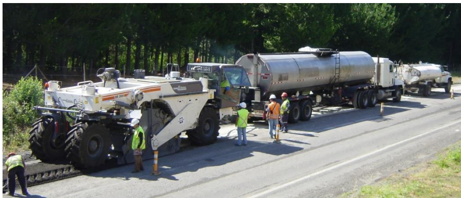
Figure 6.5 Typical Recycling Train for Bitumen Stabilisation
