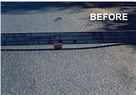
Photograph 6: Rut filling
