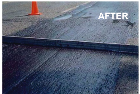
Photograph 6: Rut filling
