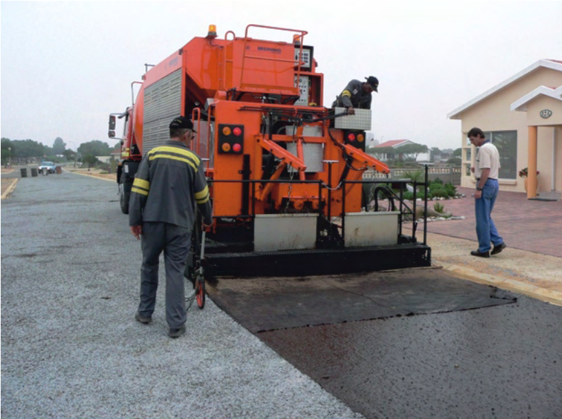
Photograph 7: Slurry overlay
