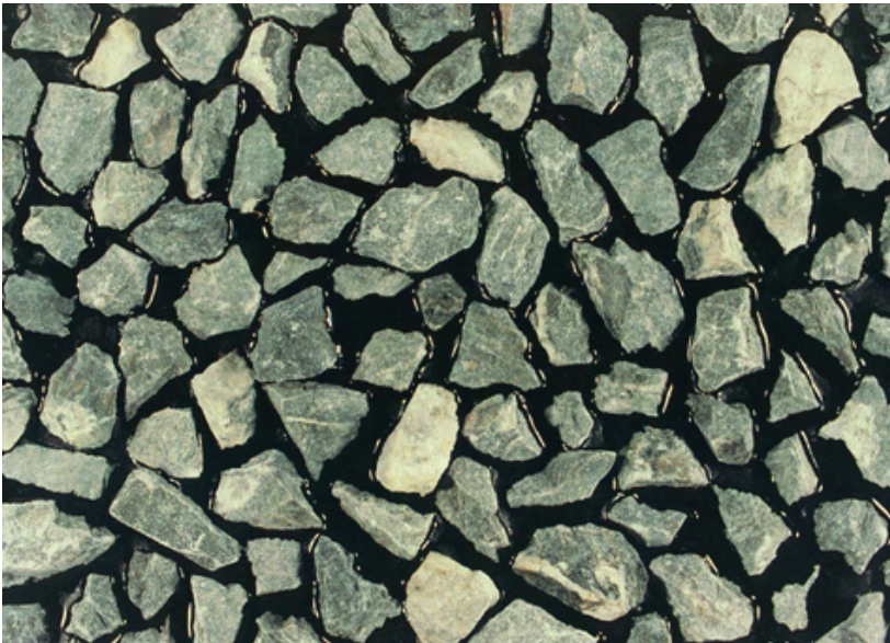
Photograph 3: Typical spread of aggregate for a Cape Seal
