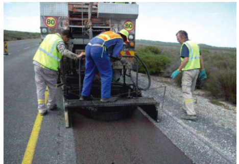
Photograph 32: Fixed width (1m) for rut fill
