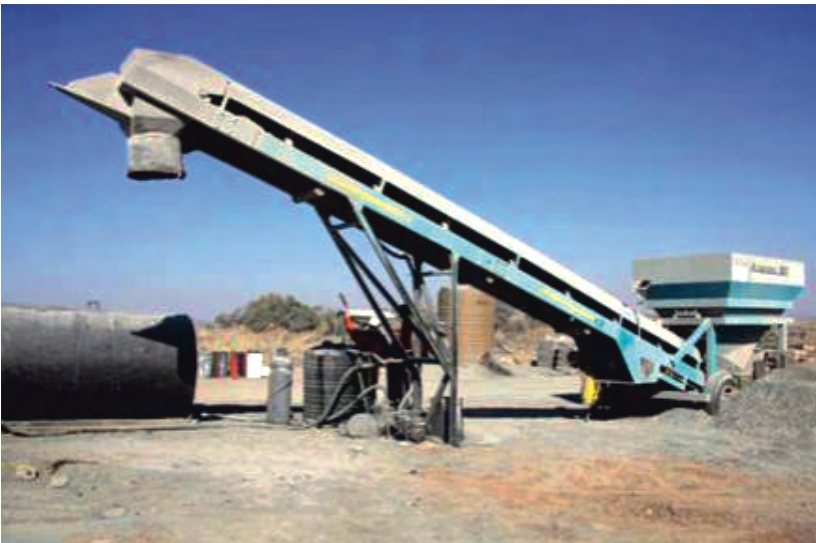
Photograph 29: Batch mixing plant
