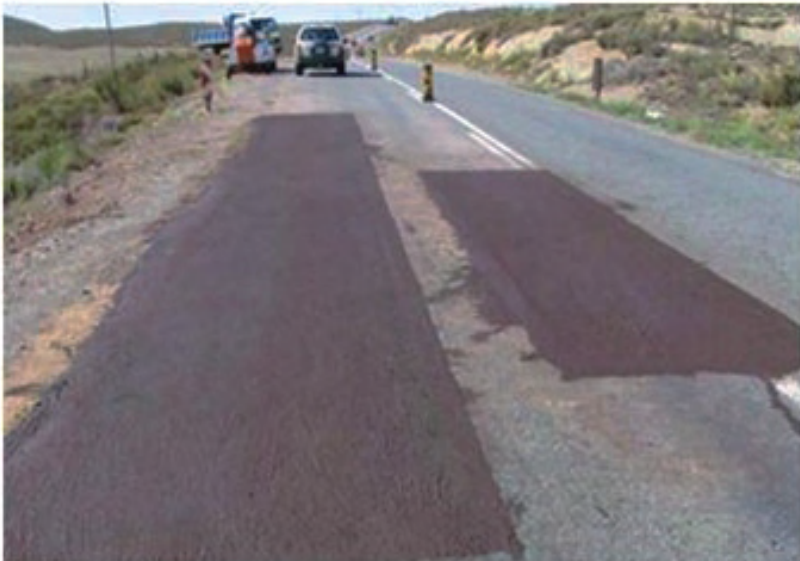
Photograph 1: Patches covered with slurry
