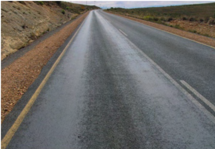
Photograph 4: Varying existing texture
