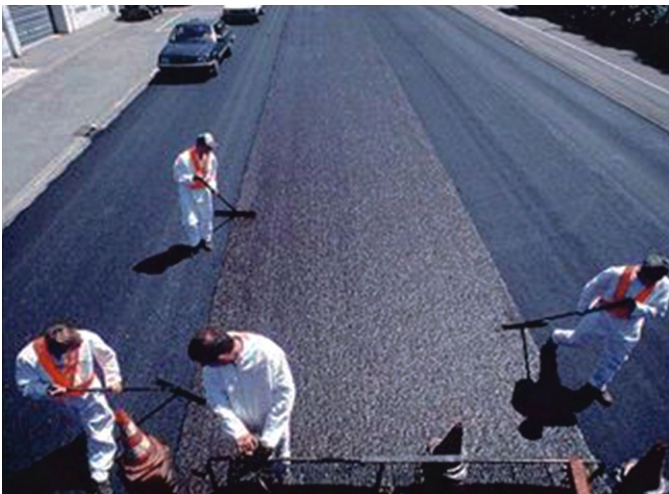
Photograph 2: Slurry as initial seal
