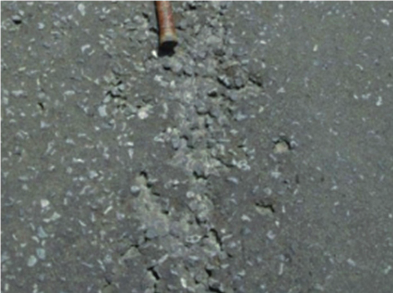
Photograph 42: Ravelling of slurry in wheel track
