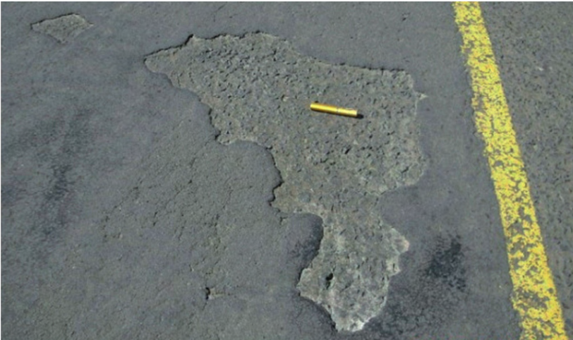
Photograph 41: Delamination
