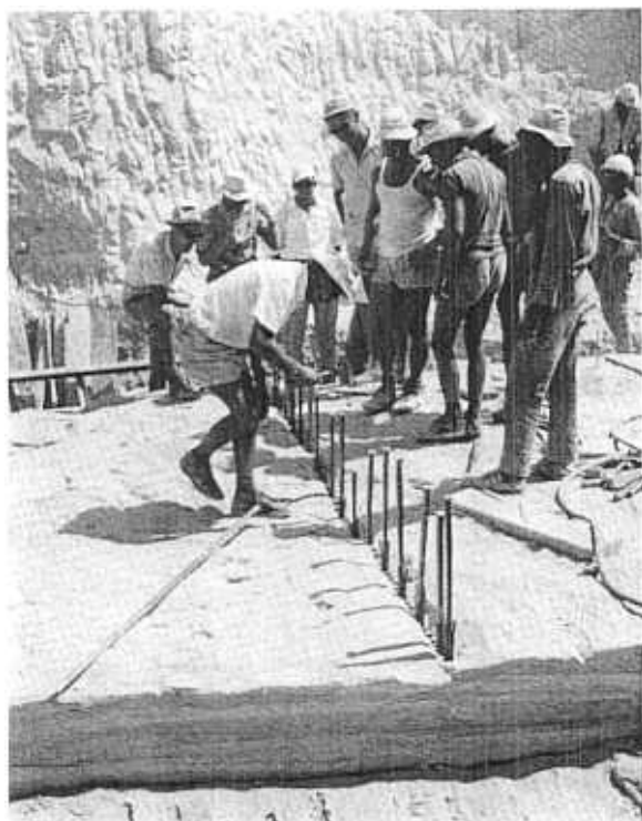
Fig. 20. - The roofs of the temple rooms were to some extent divided into blocks by boring and wedge-splitting. In this case, shallow cutting in the visible ceiling surface had to be made in advance, by means of hand-saws.
