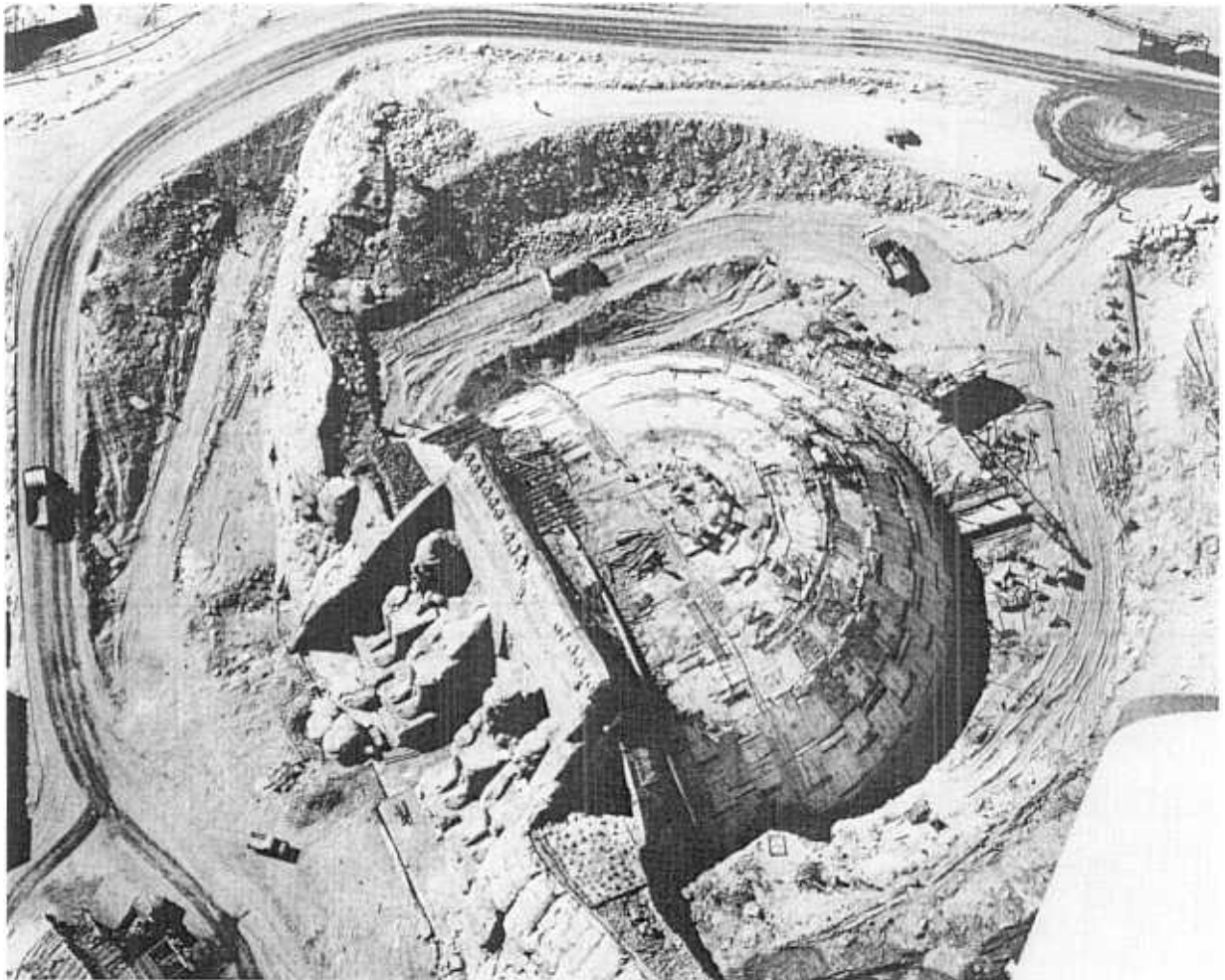
Fig. 35. - Aerial view of the Great Temple, with the re-erected façade and with the completed dome behind. The build-up of the artificial hill is the only work that remains to be done; the front stone walls have, however, already attained some height, as has also the rockfill to the rear.
