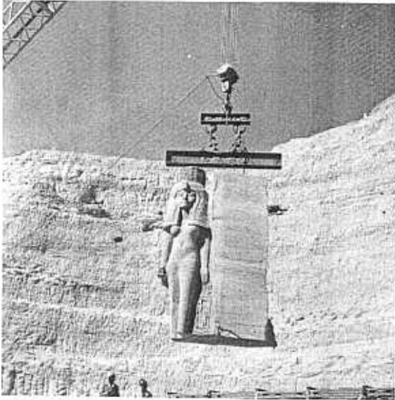
g. 22. - Queen Nefertari (Cf. Figures 4 and 5) as now temporarily loosened from her place at the leg of her royal consort. To support her slender figure, a substantial amount of rock was kept behind it in the same block.
