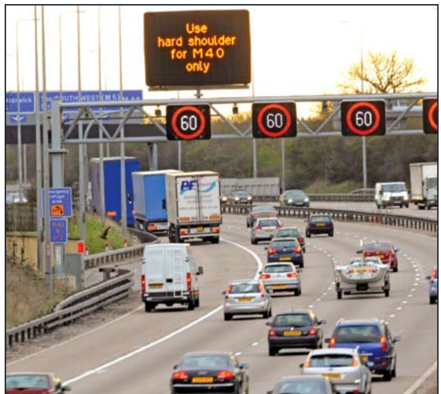
Figure 20. The use of shoulders during peak periods has become a common British congestion strategy.
