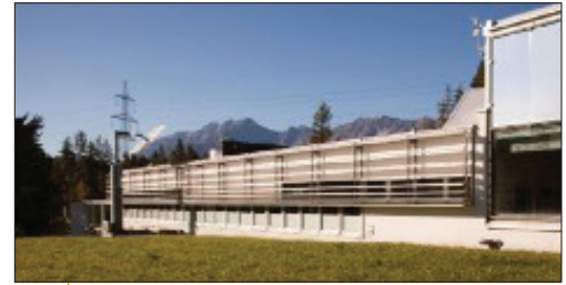
Bartenbach R&D office in Aldrans, Austria
