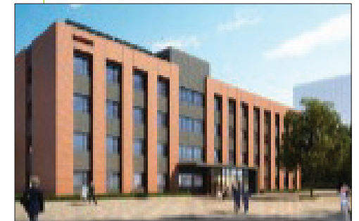
CABR NZEB in Beijing, China
