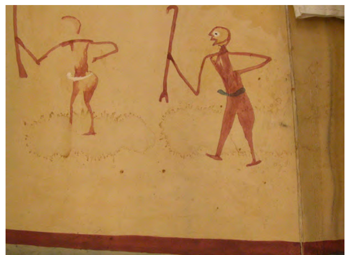
Painted Tomb problems: An example of cracking and tenting along a join as well as cockling and splash marks.
