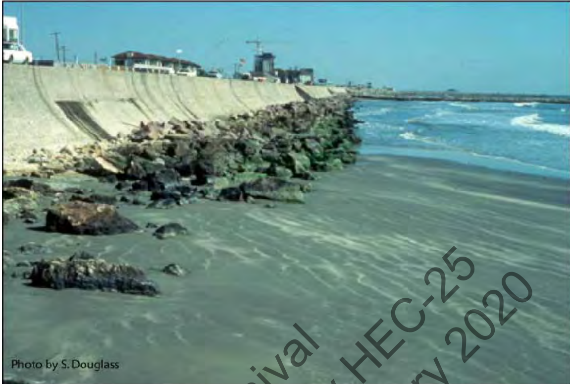
Figure 6.3. Galveston Seawall, Seawall Boulevard (1983)
