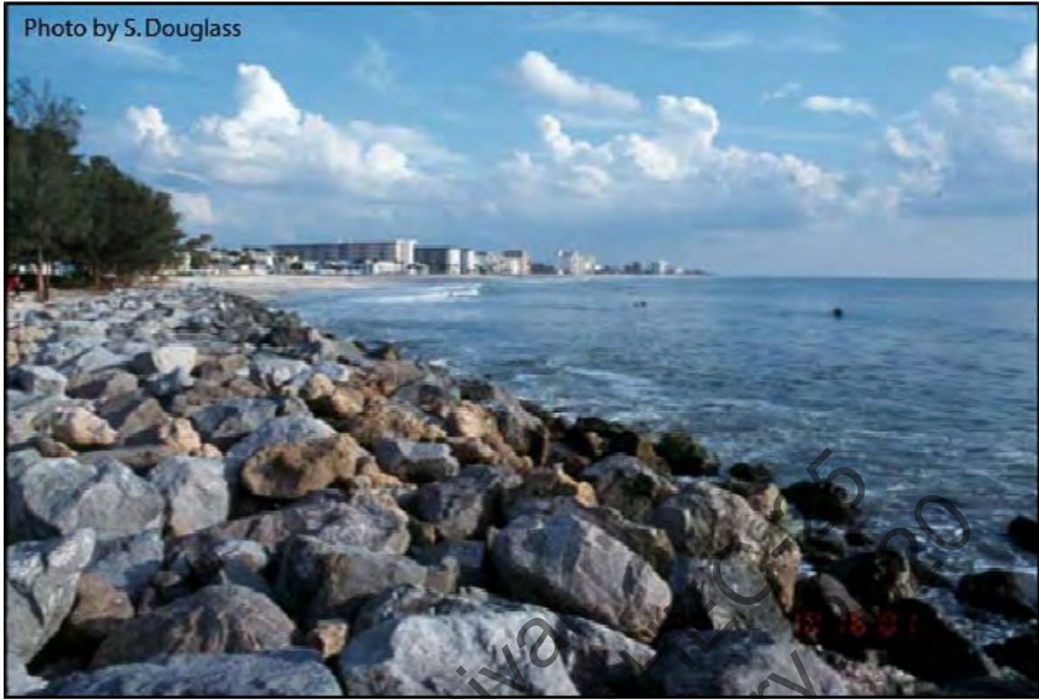
Figure 6.5. Seawall protecting a coastal highway. Venice, Florida (2001)
