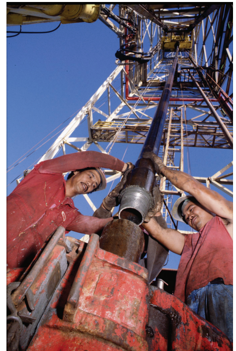
Figure 4. Making a drill pipe connection on the rig floor. The elevator (red clamp at the bottom of the picture) supports the box [or upper] end of the drill pipe and holds the weight of the entire drill string during a connection.
