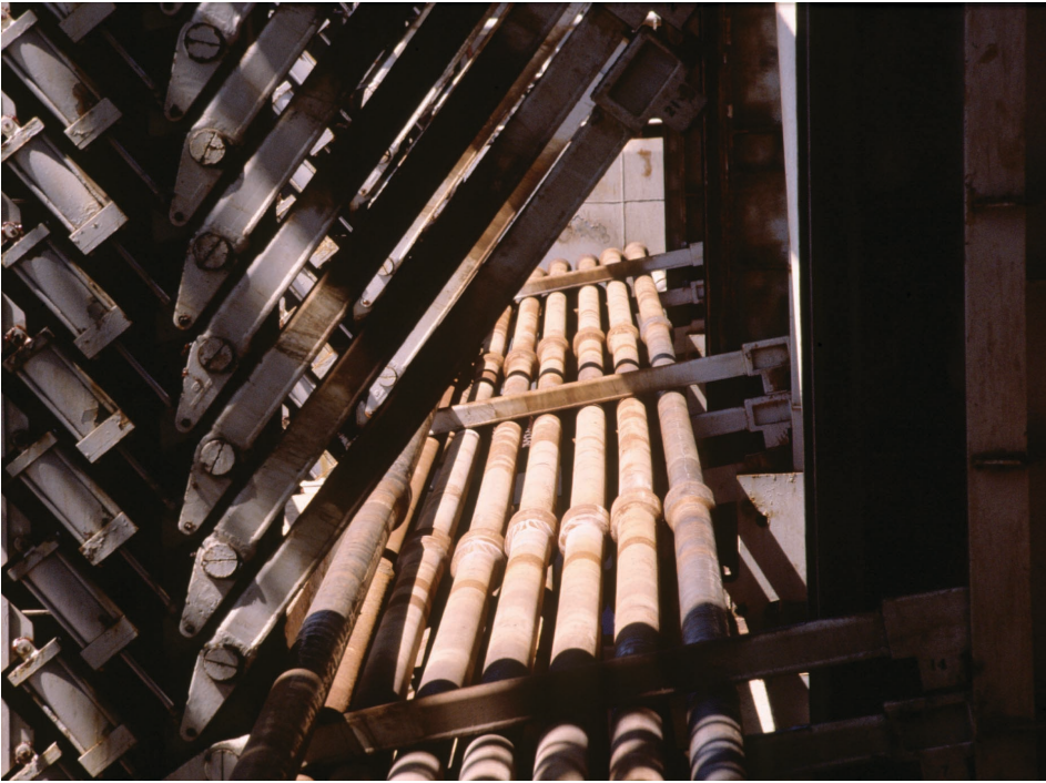
Figure 3. Drill pipe stands are stored in the horizontal pipe racker, which is located behind the derrick and rig floor.
