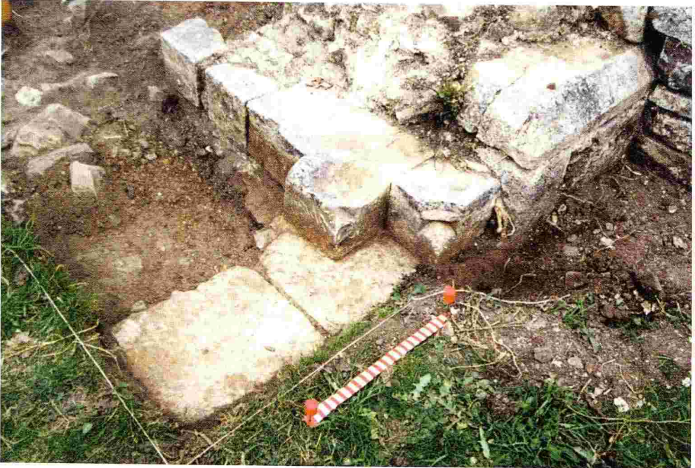
FIG. 113 – The detailed mouldings in the doorway with the stone threshold in the foreground are still in place. At the right the later stonework of the porch overlaps the plinth of the hall. This is the distinctive detail that identifies the possible master mason.
