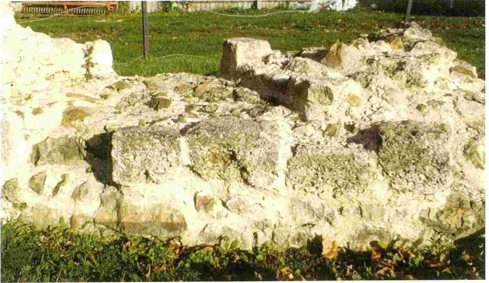
FIG. 115 - Blocks of tufa inside a window opening.
