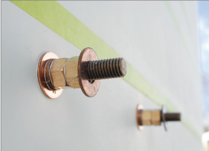
Studs on a new boat await installation of a hull anode. When completed, there should be a gap between the back of the anode and the hull.
