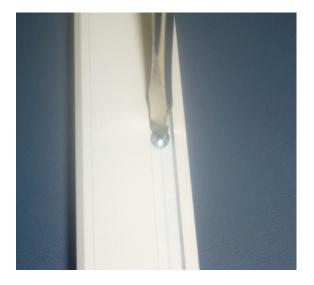
**3.** Once you have removed the screw, you are then able to adjust the fabric by sliding it back and forth (or until multi shade gap is at the desired width).
