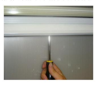
2. Remove screw in top of headrail.
