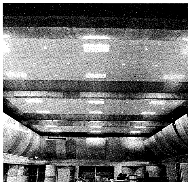
Fig. 11—One of the many combinations of adjustment possible with the three types of adjustable acoustical elements in the main portion of Studio A. These include the ceiling stepped, the middle wall panels staggered, and the wainscot panels opened at random.
