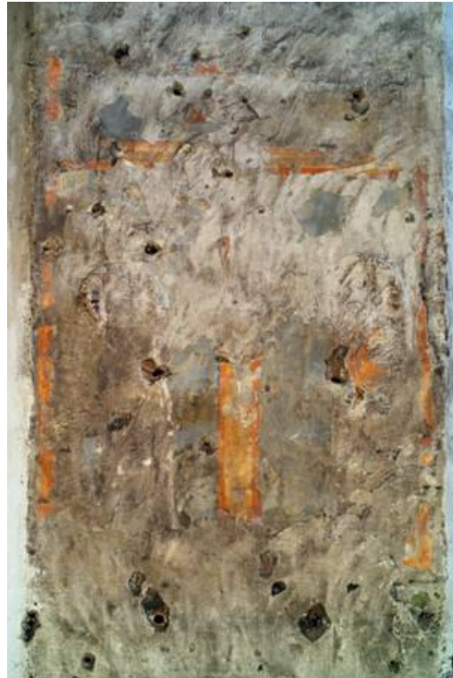
Fig.3. Fragments of composition visible in lacunae of lime-wash covering the painting. Image in visible light, scattered.
