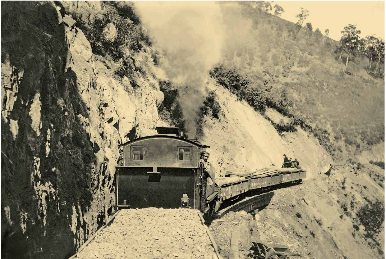
Loco 9A working bunker-first upgrade towards the photographer (and Walhalla). The three trailing NQR wagons are filled with pylons and other bridging timbers. The clearance of tree cover surely contributed to the deluge of muddy water and rocks onto the railway following torrential rains
