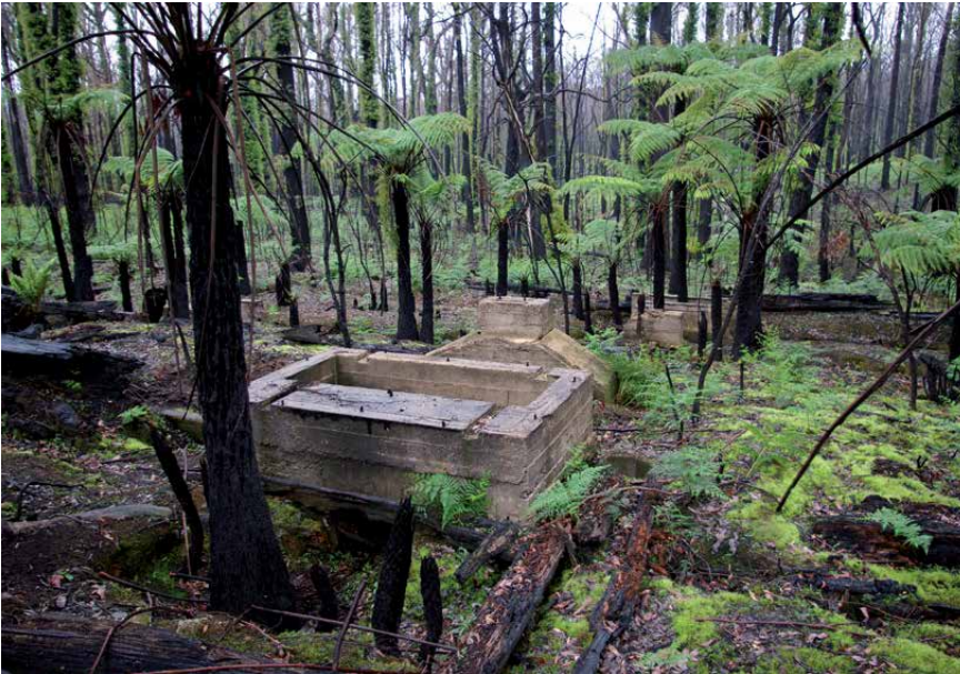
Concrete saw bench foundations looking south-east down the main sawdust trench Photo: Scott Gould
