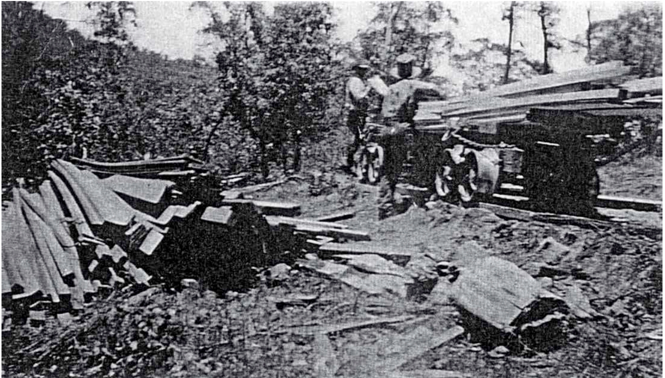
Deraillments were frequent on most Victorian timber tramways. Here, timber is being reloaded by hand onto a pair of trucks on Dumbrell's outlet tramway along Reedy Creek. Photo courtesy Nell Mildren (via Lloyd Matthews)
