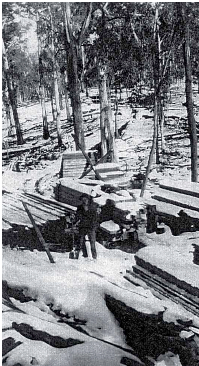
The ‘top’ mill was often snowbound in winter. Sawn timber stacked on trucks ready for its short journey north to The Gantry.
