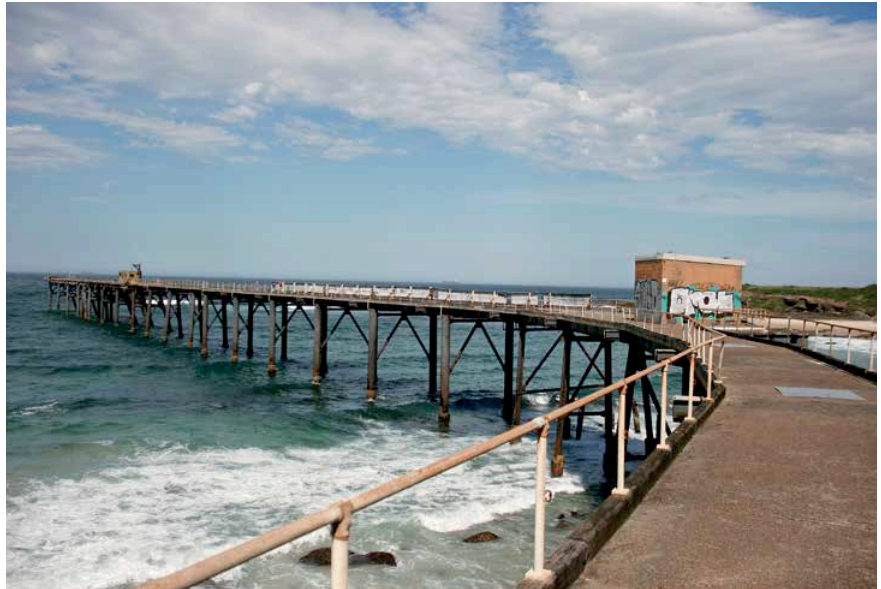
A: Looking seaward along the Catherine Hill Bay jetty with the two buildings still in situ, 21 January 2016. The curve in the foreground betrays the alignment of the former standard-gauge railway connection to the jetty. Photo: Sohtaka Kikuchi
