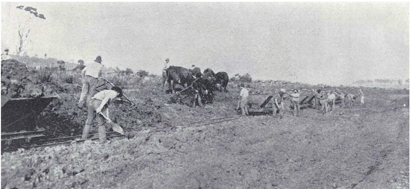
An interesting pair of photographs, taken a few minutes apart. In the top one a bullock team is approaching the camera, breaking the earth with a large single-furrow plough. The shovel-men are on the high side of the track, loading the broken earth (from the plough's previous pass) into side-tipping skips. The loco can just be seen at the far right. In the lower picture the plough has passed behind the photographer, and crossed to the high side of the tramline and is breaking the earth. The shovel-men have swapped to the lower side and are shovelling the latest lot of loosened earth into the skips. When full, the loco will bring back the other set of emptied skips, and collect the lot in the the photos. Judging by the loaded skip at the left, the loco is overdue! When the easier-to-work upper soils had been removed, a Ruston Proctor steam-powered shovel was introduced.
