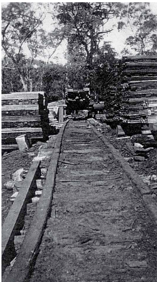
Timber chocked ready for loading onto trucks on the export tramway leading from the top mill to The Gantry.
