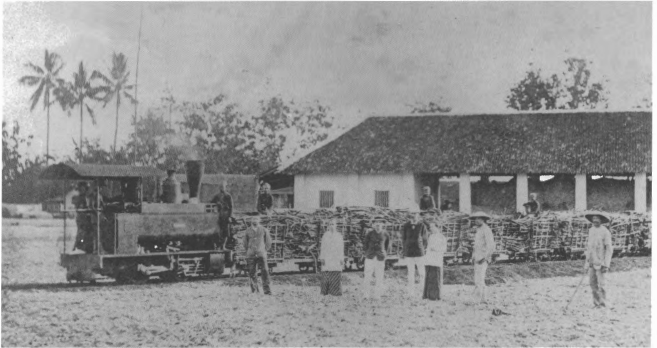
CSR records include this photograph of Decauville's eighth locomotive, PANGKA (Couillet 576 of 1882), a 5½ ton 600mm gauge locomotive, delivered to a sugar mill at Pangka in Java. Note that the locomotive has pannier-style tanks and that the cane is loaded on the trucks longitudinally. The neat building construction and manicured surroundings are in contrast with contemporary Queensland scenes.
