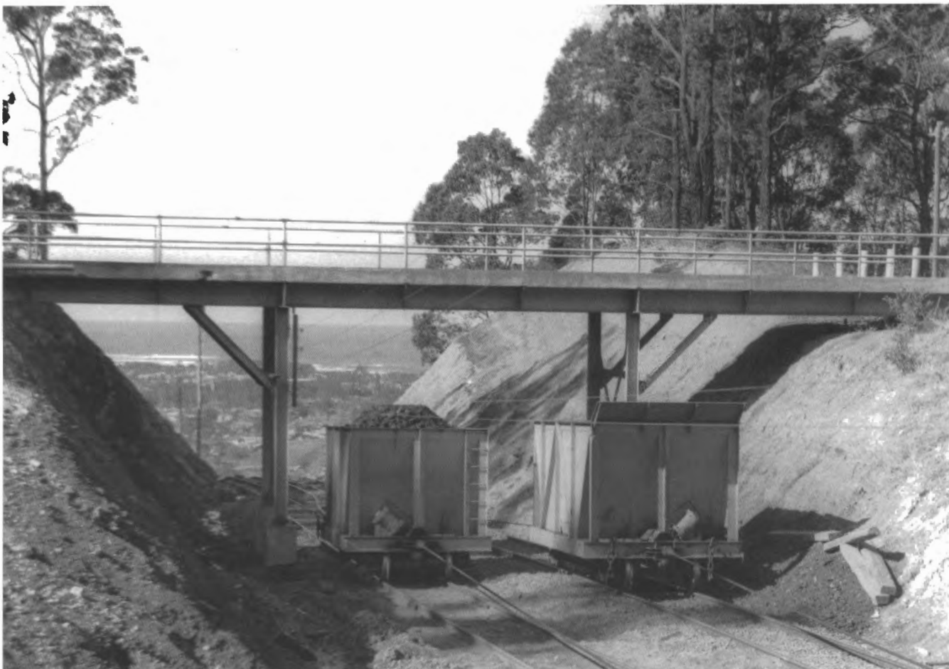
In 1956, a new incline was built to take the coal from the mine to the screens on the coastal plain. Again working on the self acting principle where the descending loaded hopper hauled its empty colleague back to the top, the system used track of 3ft 6in gauge, thus introducing the third dimension used at Corrimal. The incline was single track with the hoppers passing at a mid-way loop. Photo: Ron Preston
