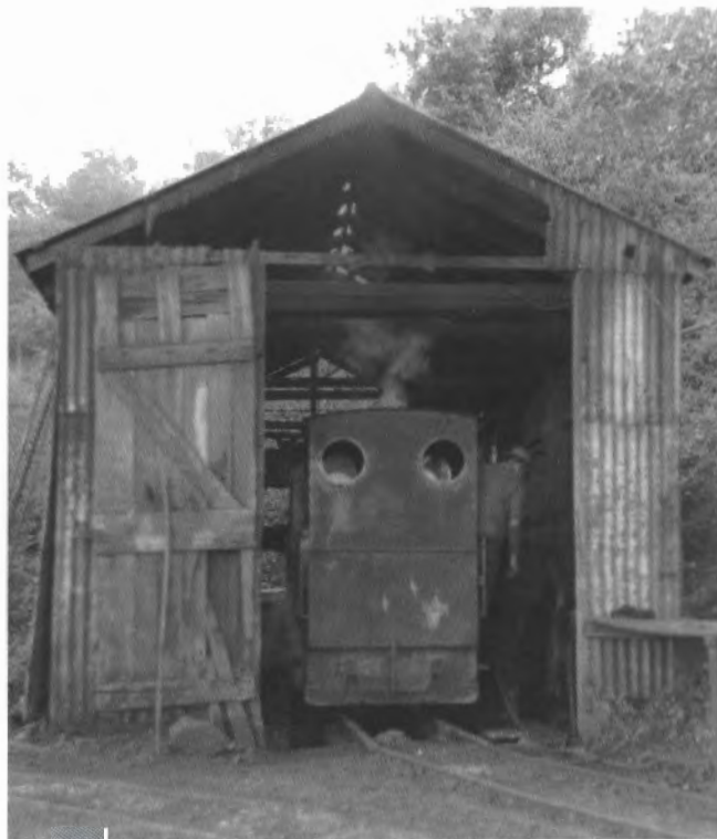
A tiny engine shed was provided near the mine entrance and within the iron and timber structure, BURRA and the Robert Hudson loco were stabled. Beneath the rails, a small pit allowed the long-suffering maintenance staff access to the valve gear, ash pan, brakes and other complexities of the small locomotives. Photo: Ron Preston
