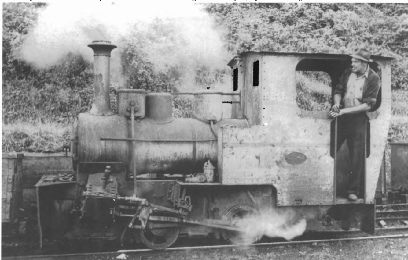
The last member of the narrow gauge fleet was this 0-4-0 well tank, originally supplied by Robert Hudson to National Portland Cement Co. for their Maria Island plant, off the east coast of Tasmania, in 1922. The 5.6 ton engine came to Corrimal in 1944 to replace Krauss 6927 of 1914. The driver, taller than the diminutive cab, looks along his train of four-wheel skips before heading another load across the mountain to the incline.
