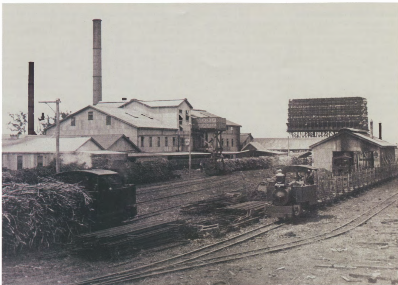
Childers Mill, circa 1910. Fowler 0-6-2T number 5 (11223 of 1907) arrives from the west with a trainload of wholestick cane, while in the background one of the second pair of Fowler 0-6-0Ts, number 2 (7606 of 1896) or number 3 (7607 of 1896) brings a loaded train in from the east. In the foreground, the other 1896 Fowler 0-6-0T brings a train of empties past the loco shed, while ex-Knockroe Mill Decauville 0-6-2T TORPEDO (245 of 1897) sits outside.
