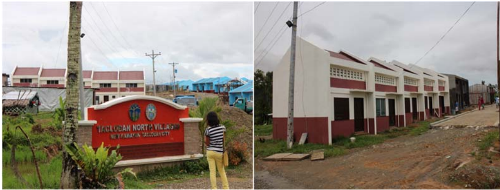
Fig. 11-12. In the same North Tacloban resettlement site there are also houses built by Habitat for Humanity
