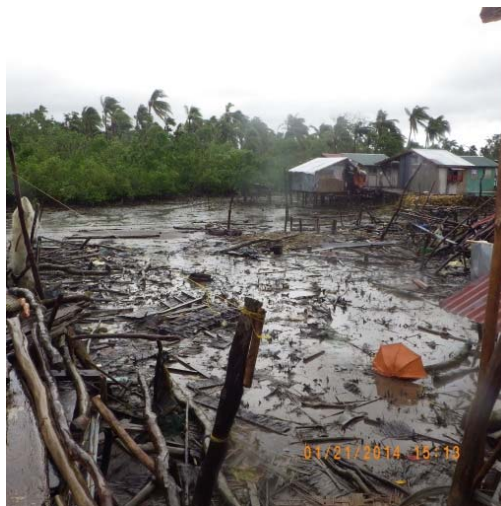
Fig.5-26. Damage in Quinapondan fishing village.
