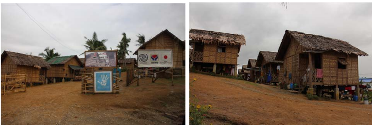
Fig. 11-9. Transitional Shelters in Tagpuro, in the north part of Tacloban City, Feb 2015
