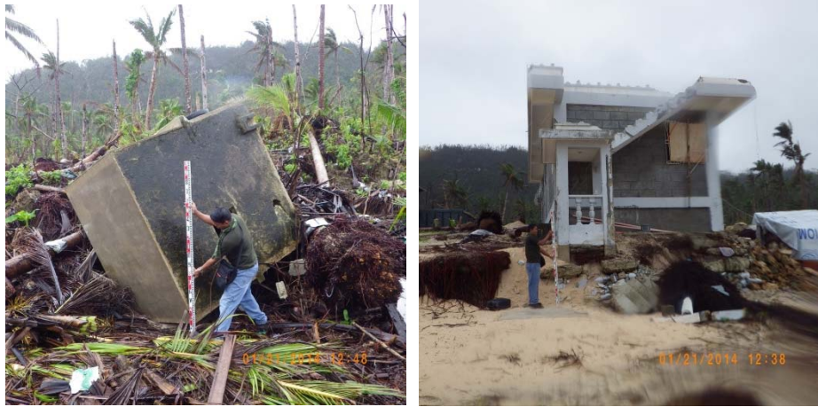
Fig.5-24. Damage in a coastal Barangay of Salcedo. Toilet vault (left) deposited on land at 9 m above Mean Sea Level. (right) top story at 11.6 m above Mean Sea Level washed away.
