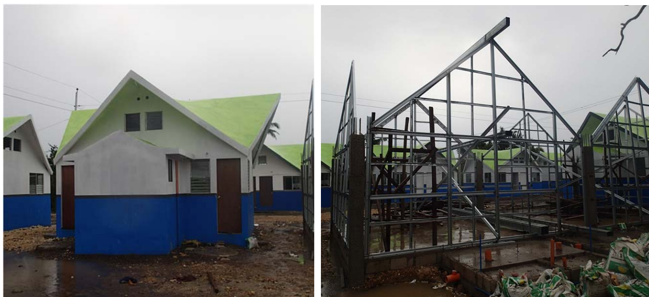
Fig. 9-16. Permanent houses provided by UN-Habitat in Daanbantayan, Cebu
