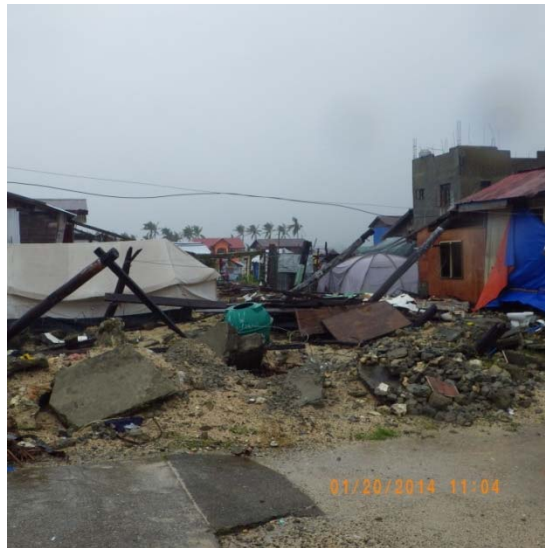
Fig.5-28. Piles of house washed away by bore-like surge in Hernani.
