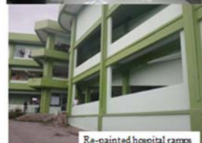
Re-painted hospital ramps
