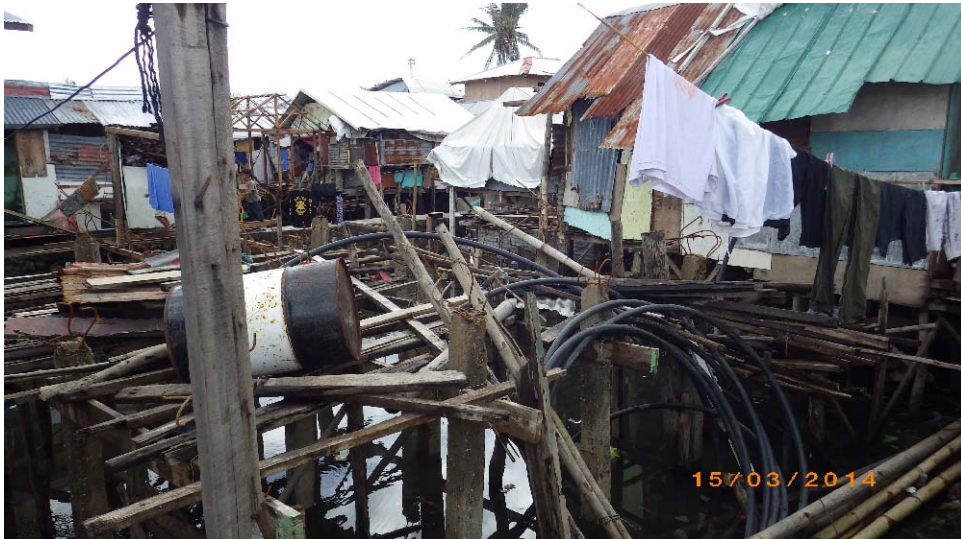
Fig.5-16. Corrugated Galvanized Iron (GI) sheet roof for residential house commonly found in Tacloban Area.
