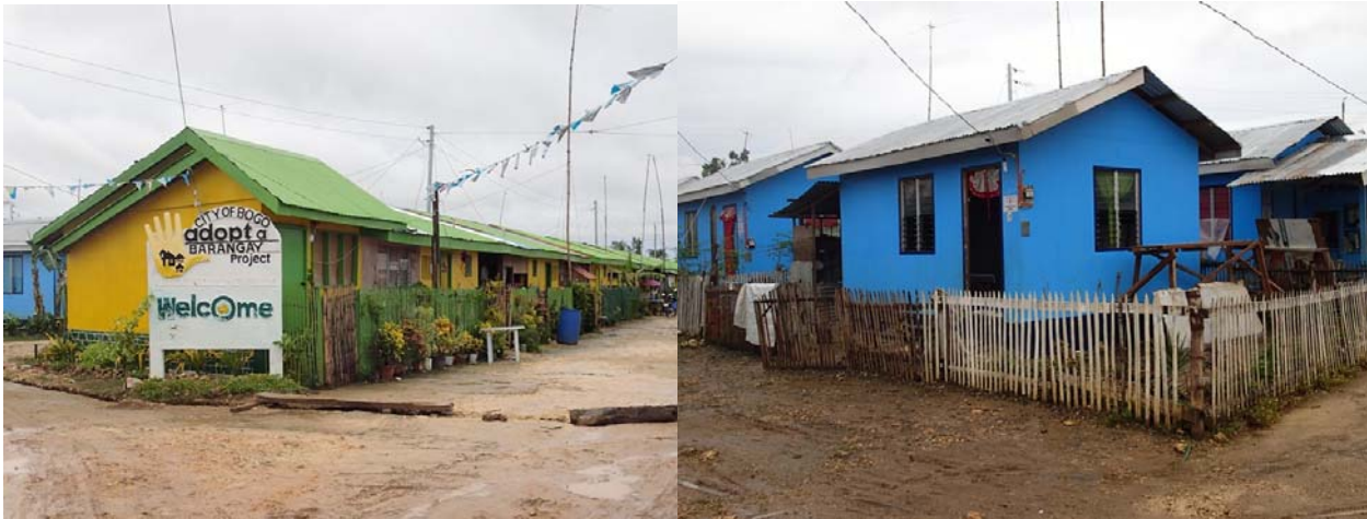
Fig. 9-17. Permanent houses located in Bogo city, Cebu
