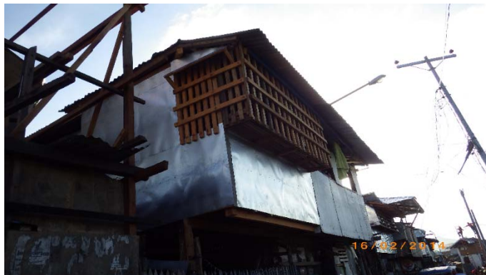
Fig.5-10. A partially damaged house reconstructed its outer wall in downtown Tacloban.
