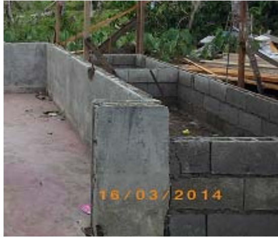
Fig.5-9. Brick house wall with few longitudinal reinforced wire
