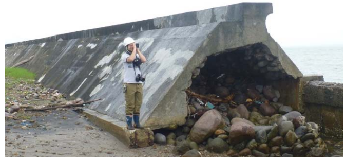
Fig.5-30. Seawall breach on eastern coastline of Tacloban Airport. Crest height 3 m above Mean Sea Level.
