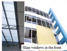
Glass windows in the front
