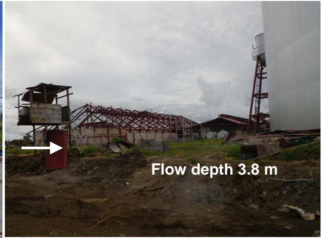
Fig. 12-6. 3.8 m depth of inundation measured at 120 m inland along the Tolosa transect.
