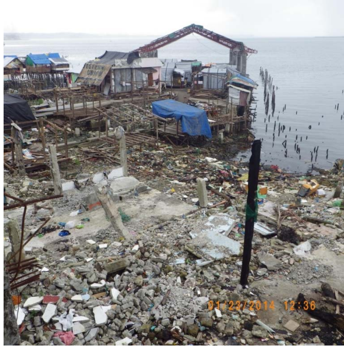
Fig.5-12. Destruction of Reinforced Concrete building in coastal downtown Tacloban.
