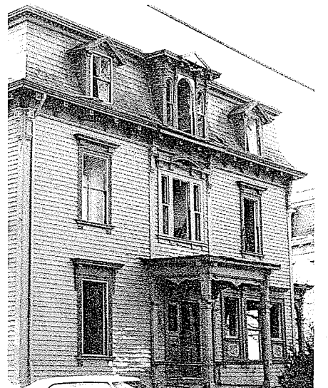
Providence buildings like this are being considered for substantial rehabilitation.
