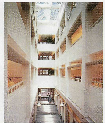
Morgan Hall. Staff space is organized around lightwells that allow daylight to penetrate the building. The skylight's efficiency is boosted by computerized rotating mirrors.
