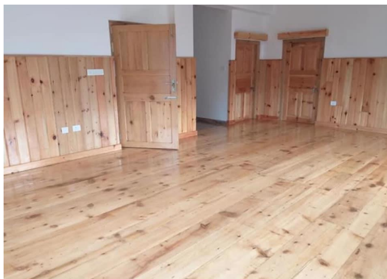
Planks on concrete
