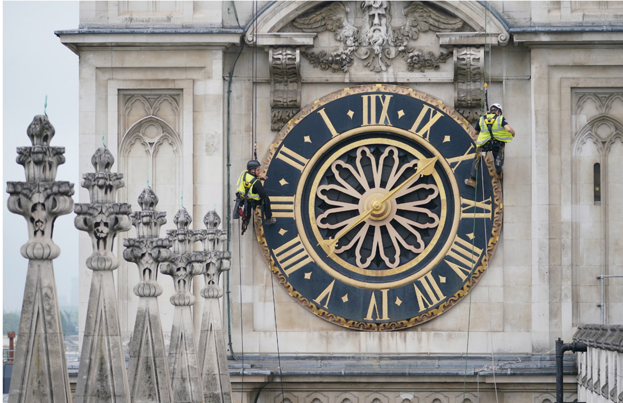
Specialist abseilers carry out an inspection of the Abbey's West Towers in September Picture: Yui Mok/PA Wire
