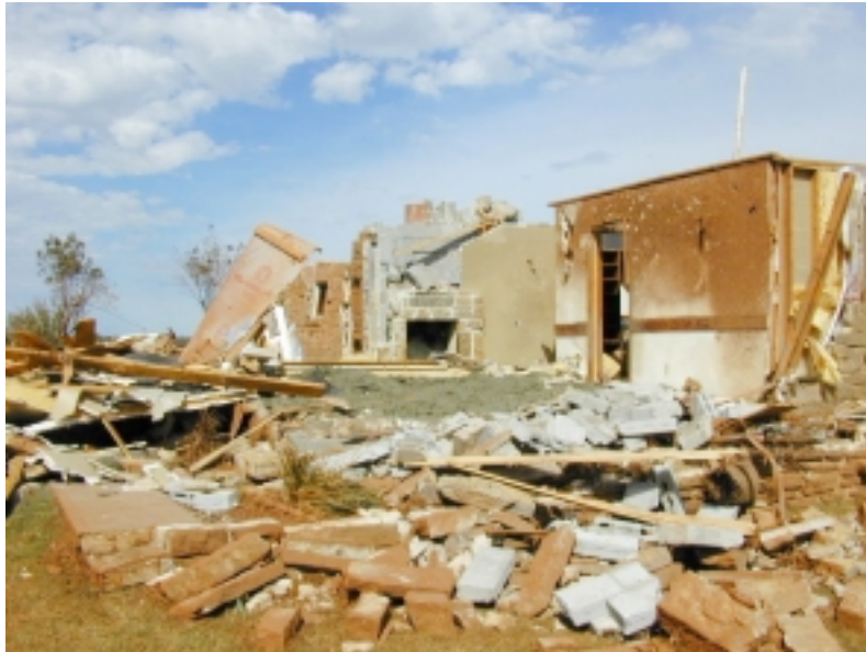
A home in southwest Custer County that sustained F3 damage.
