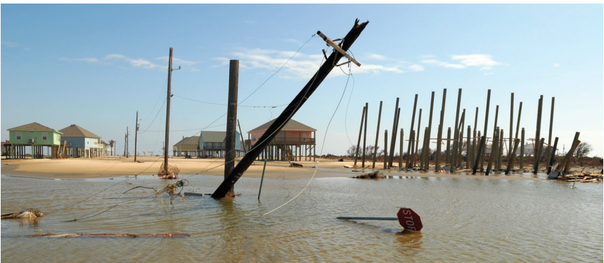
Bolivar Peninsula, TX, September 20, 2008: Damaged houses, debris and downed power lines resulting from Hurricane Ike. Photo by Jocelyn Augustino, FEMA.
