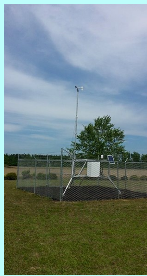
Conway RAWs after installation
