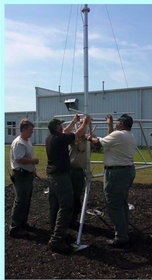
SCFC foresters installing the anemometer on the Conway RAWs
