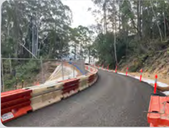
Tyalgum Road and Reserve Creek Road land slip repair updates
