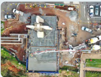
Captain Cook Lighthouse at Point Danger redevelopment
