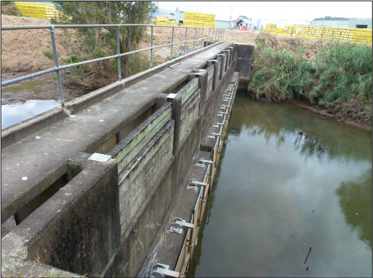
Plate 1 Flood Gate 17L (Condong Creek)
