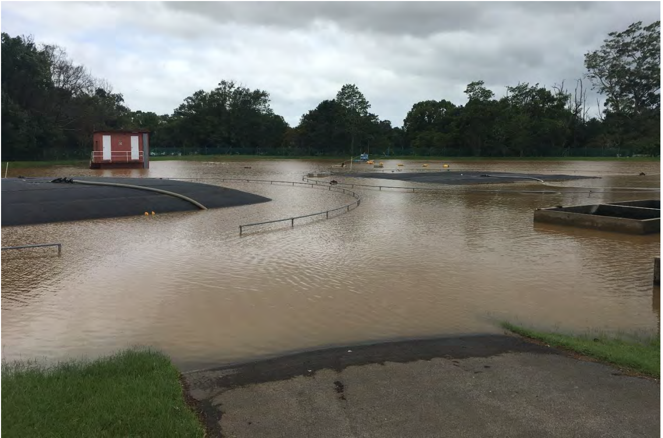
Murwillumbah Sewage Treatment Plant (1:30pm on 31 March 2017)
