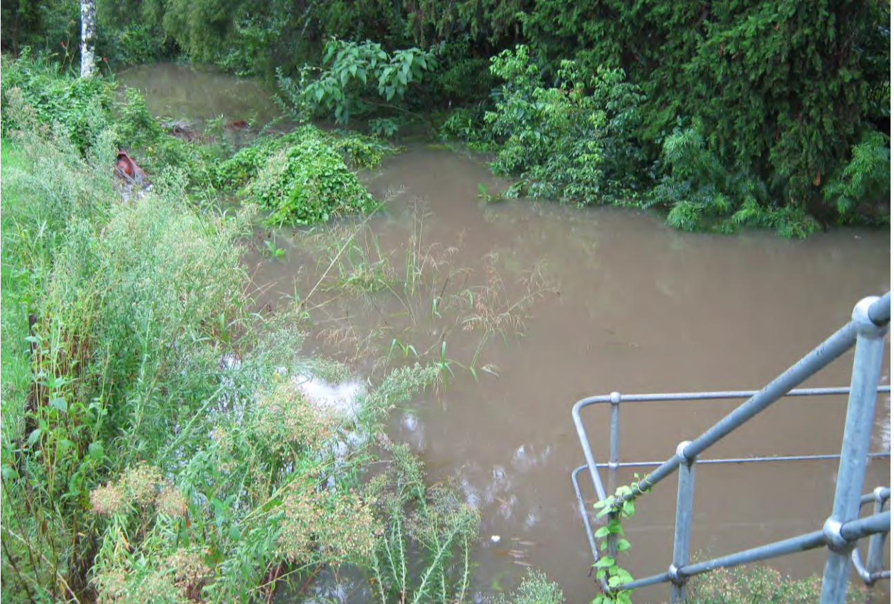
Upstream of Lavender Creek Pump Station
