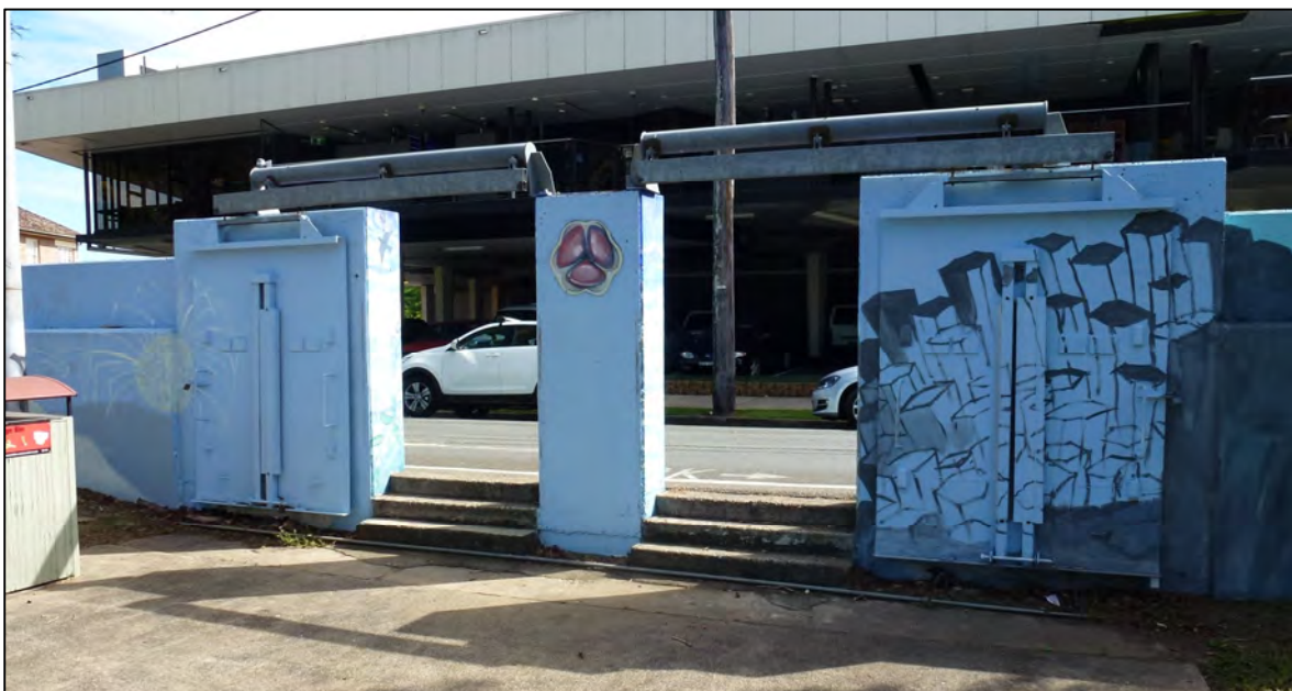
Plate 2 View looking west towards Murwillumbah Services Club showing concrete panel section of the Commercial Road levee with gated openings
