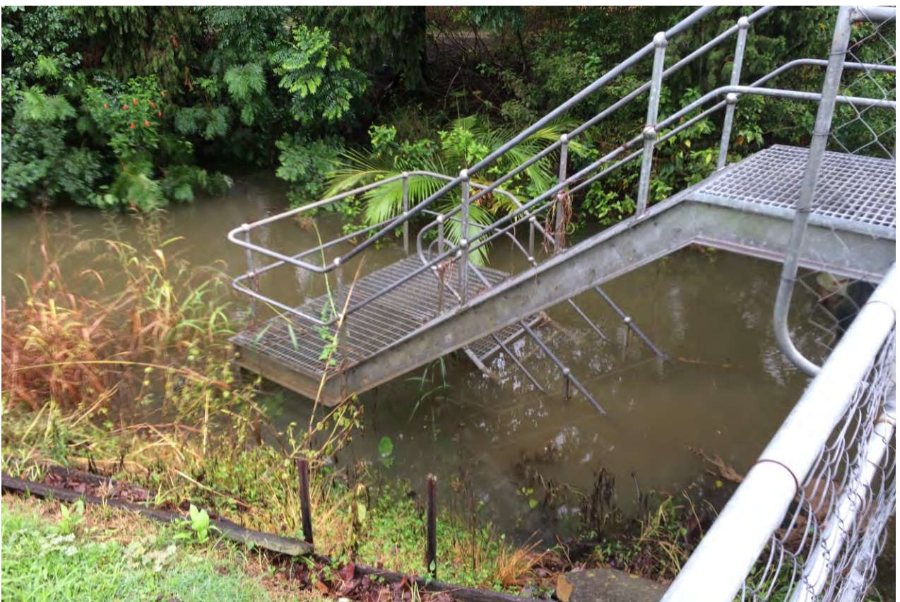
Upstream of Lavender Creek Pump Station
