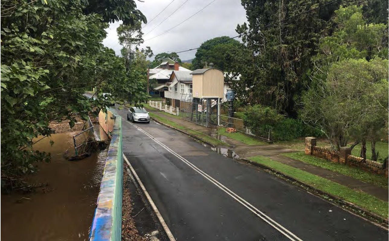
Lavender Creek Pump Station (9:00am on 31 March 2017)
