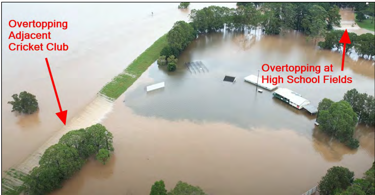
Photo 6: CBD Levee overtopping near Cricket Club and High School ( https://www.youtube.com/watch?v=UsPF5DTI44U )
