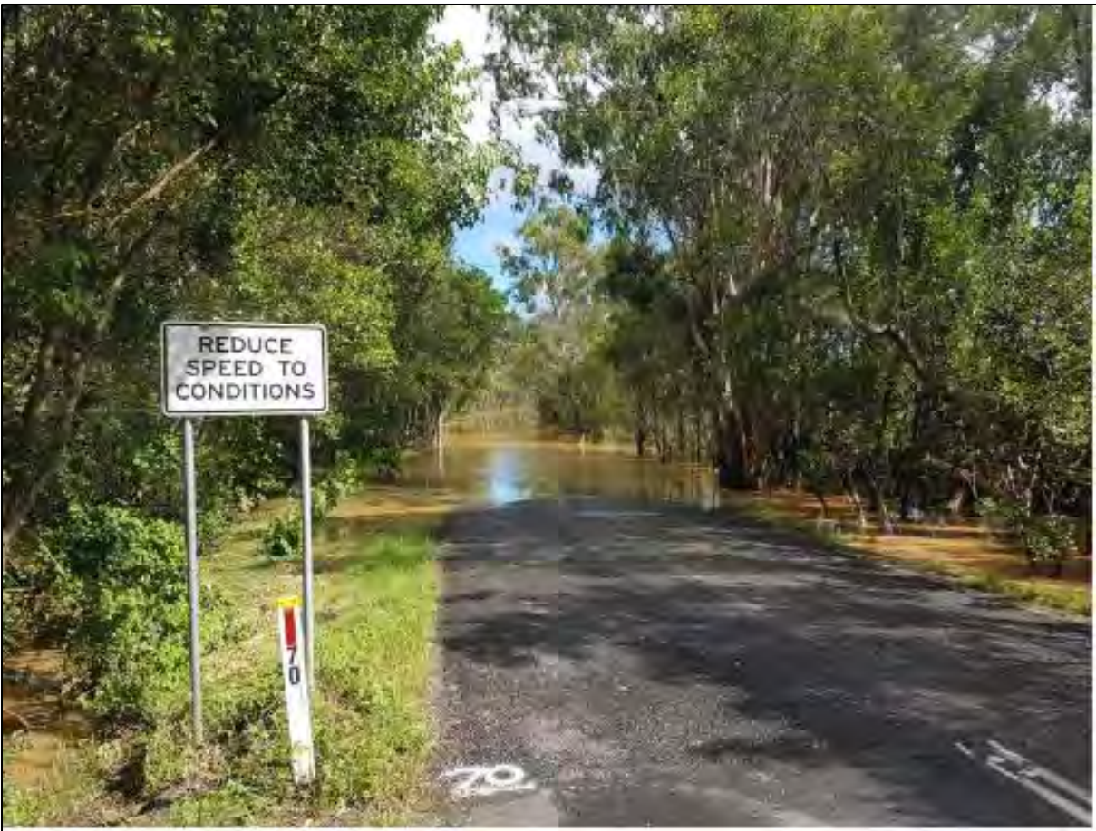
Photo 10: 2/03/2022 at 09:30 Piggabeen Road near Cobaki Road
