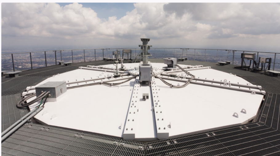
頂部避雷針(634m部分) Pinnacle lightning rod (at 634m)
