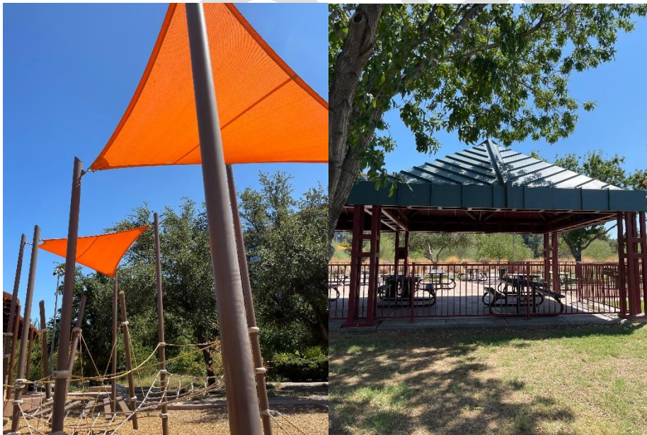
Figure 20. Shade structures at Margaret T. Hance Park
