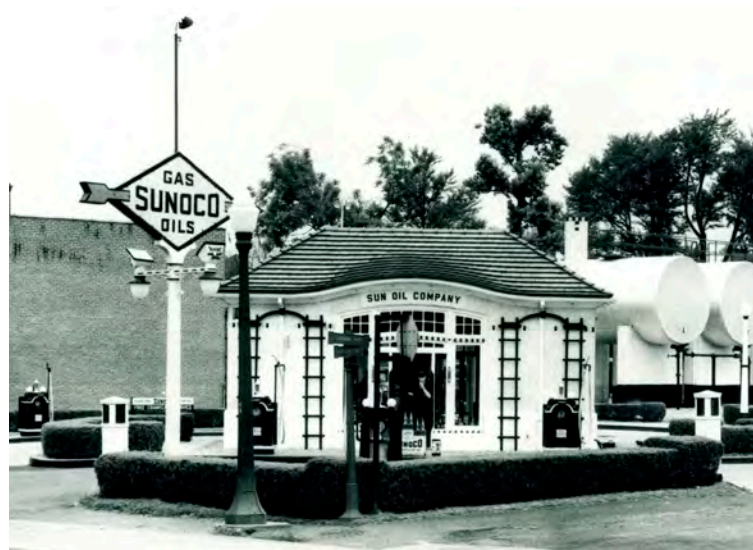
The first Sunoco service station was in Ardmore, Pennsylvania. Sun Oil Co. was an innovator in developing gasoline that was less expensive and less harmful to the environment. The Hagley Museum and Library
