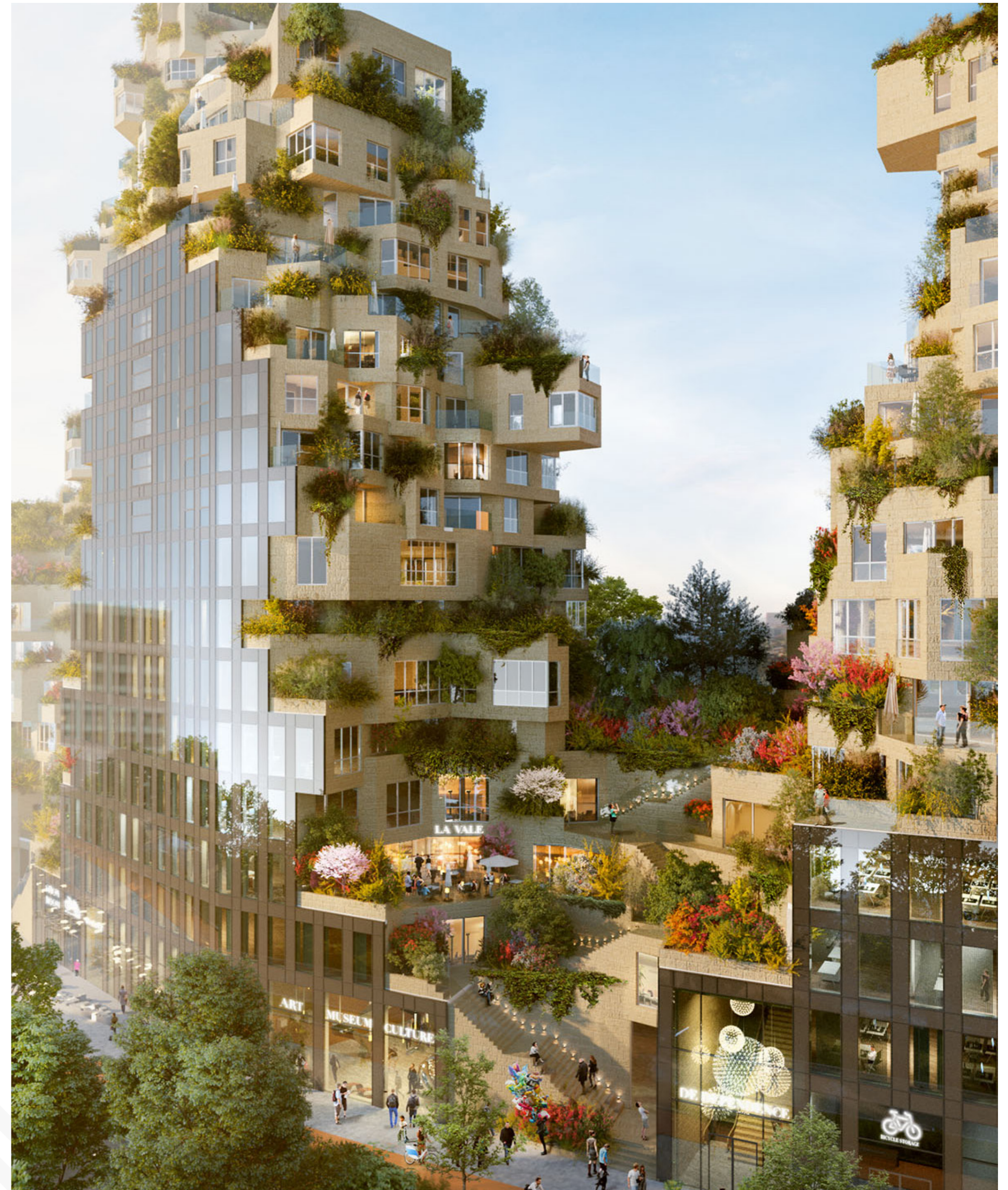
The Valley, the new home of Palo Alto Networks Amsterdam
