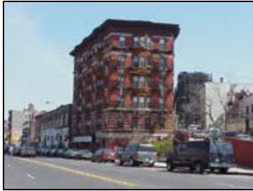
Six-story multi-family building with storefront house of worship.
