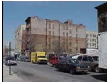
Vacant five-story multi-family building at East 166th Street between Third and Washington Avenues
