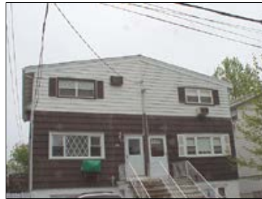
Shallow-pitched roofs on new semi-detached development
