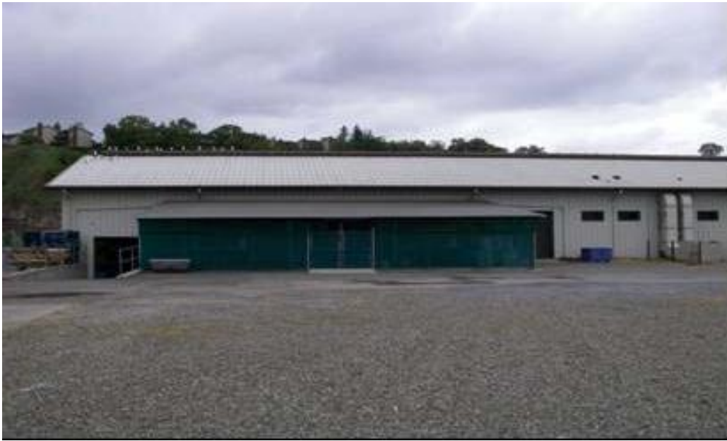
Figure 4-12. Exterior of NFH Building 2.
