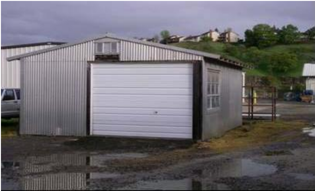
Figure 4-29. Lawn Equipment Building.
