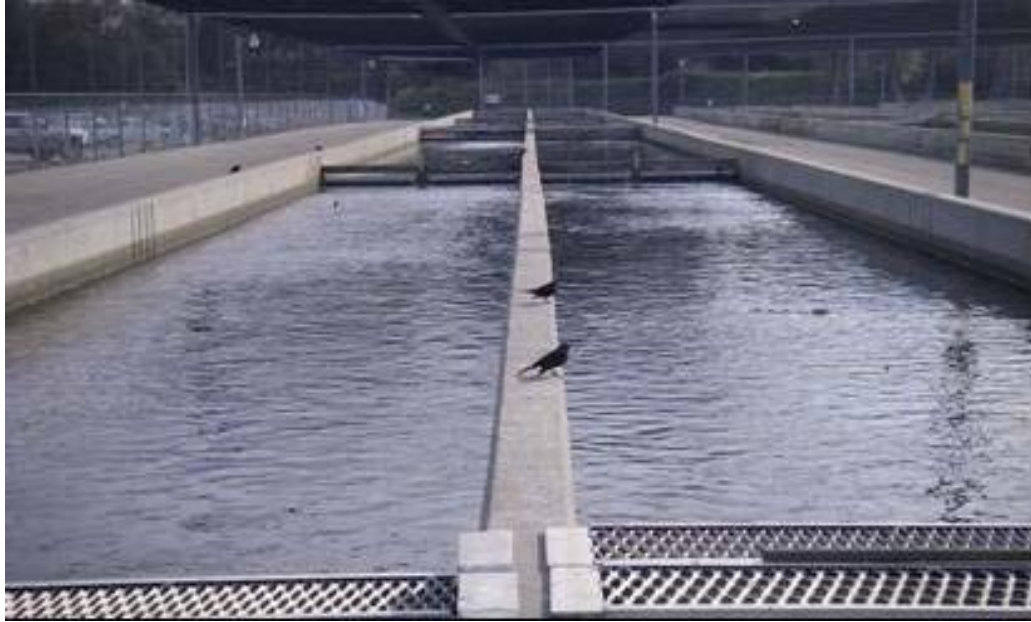
Figure 4-20. Concrete raceway ponds facing north.
