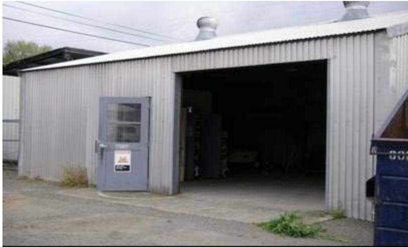
Figure 4-31. Equipment, Paint, and Fuel Storage Building.
