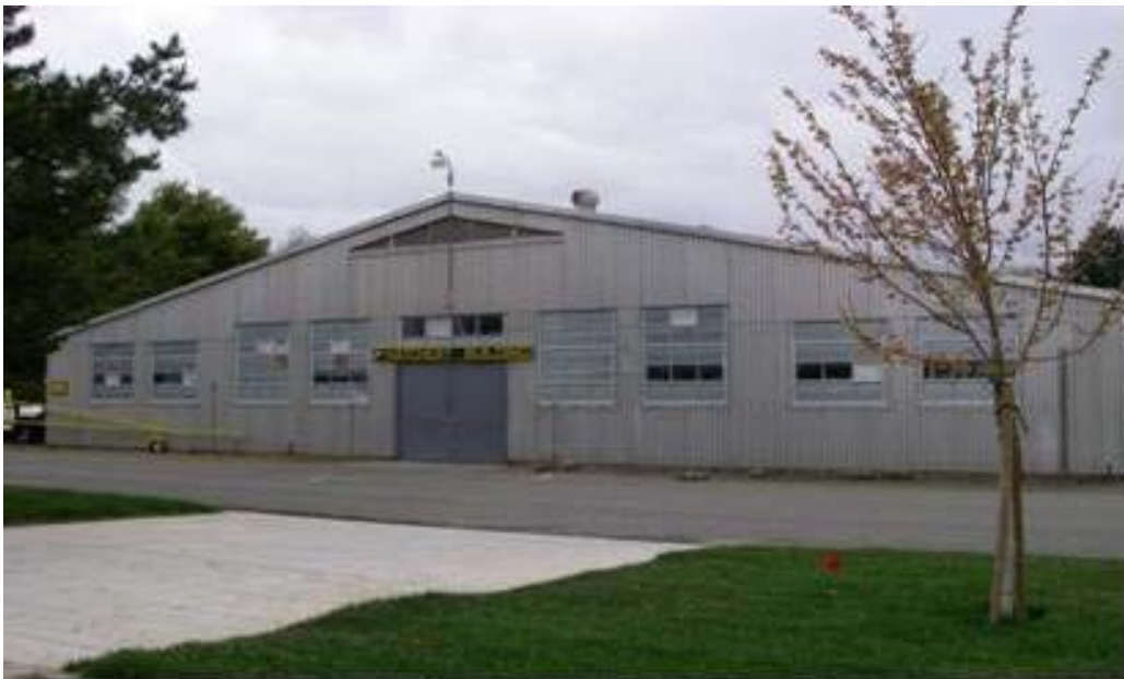
Figure 4-17. Exterior of NFH Building 1.
