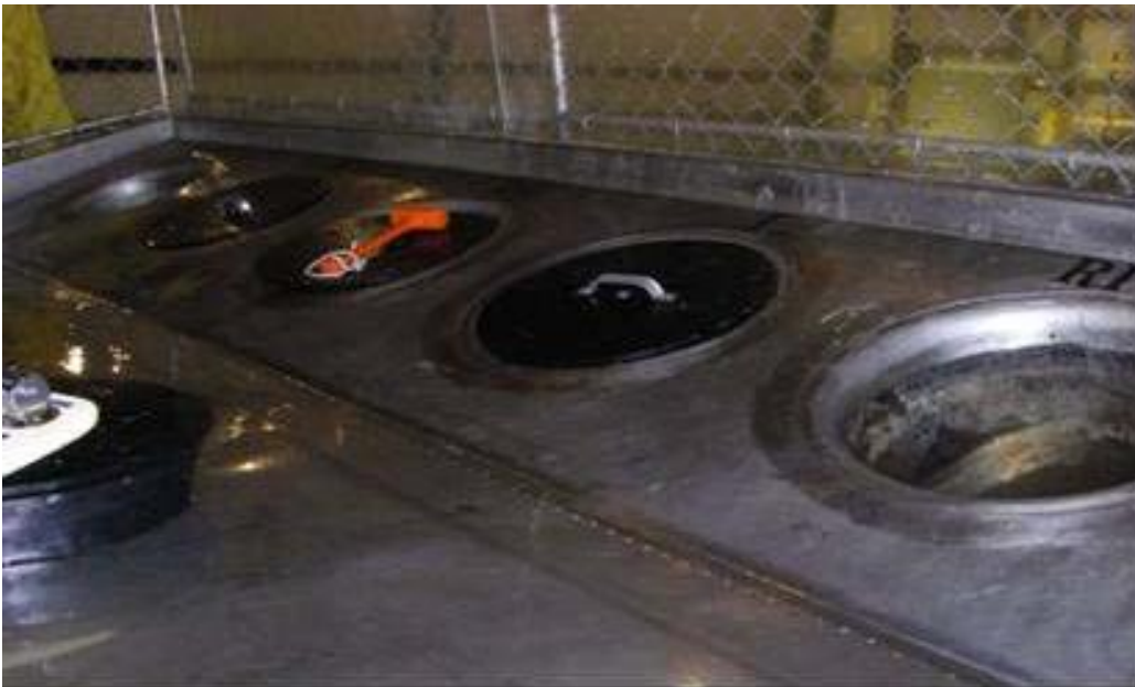
Figure 4-11. Stainless steel tubes that lead to either the holding ponds or the river.
