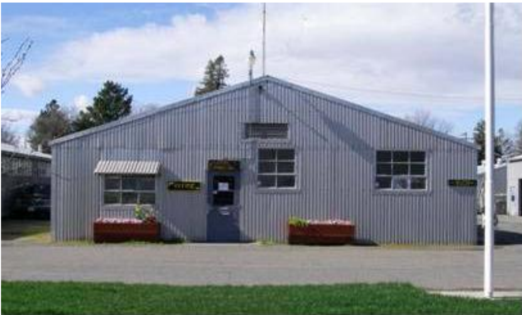
Figure 4-25. Exterior of the Fish NFH Headquarters/Office Building.
