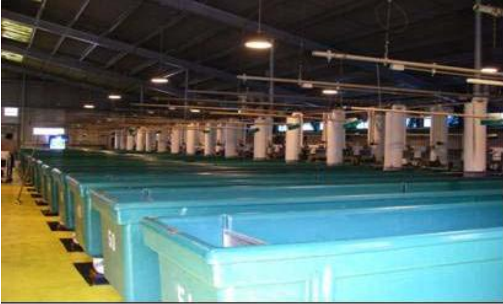
Figure 4-18. Interior of NFH Building 1.
