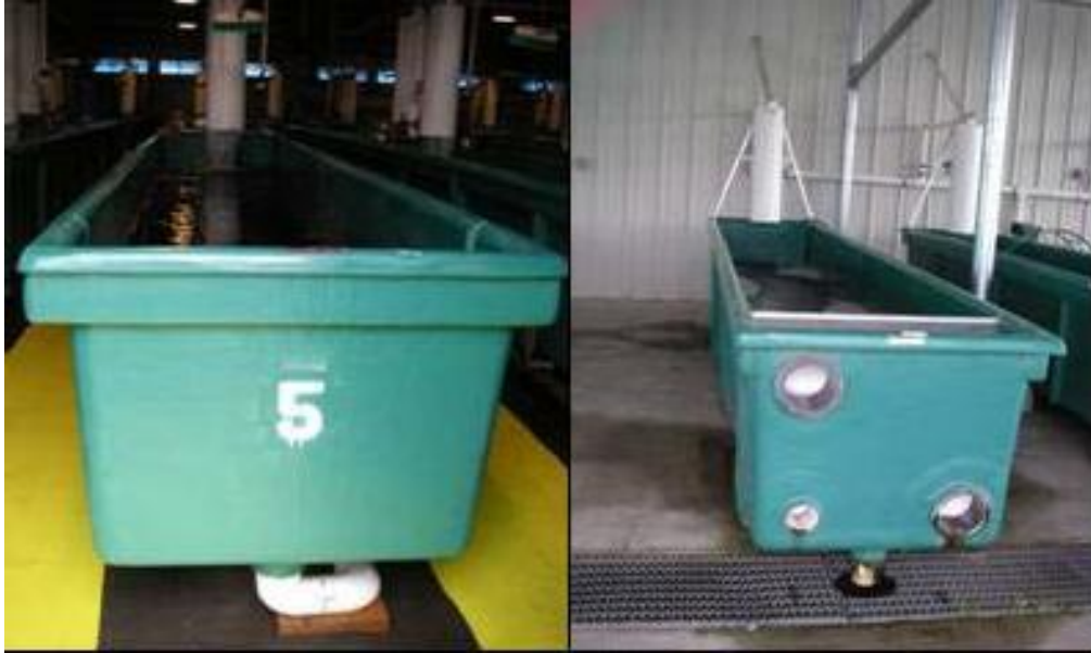
Figure 4-14 Fiberglass deep tanks used in NFH Buildings 1 and 2.
